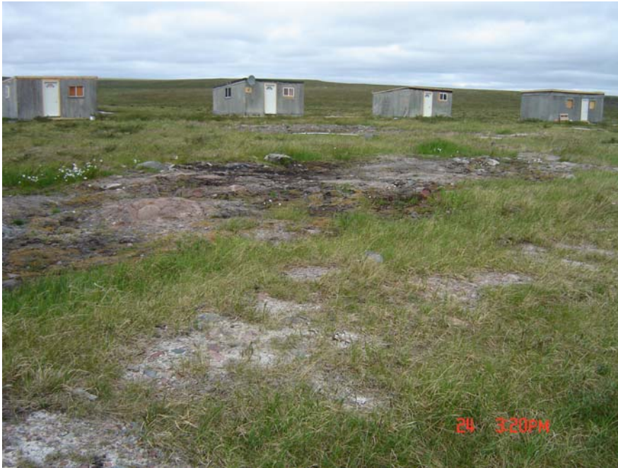
Example of surface disturbance from an old building that was removed in 2003 and 2004. Reclamation options are being investigated.
