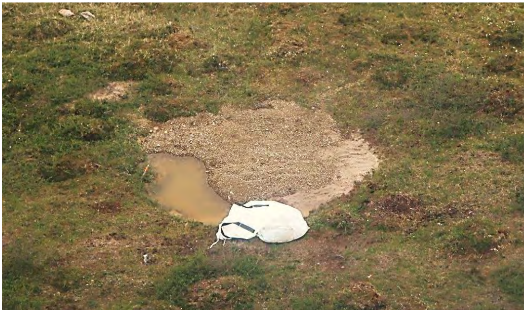
Photograph 3.7-4: Filling Sink Hole at EE-05
