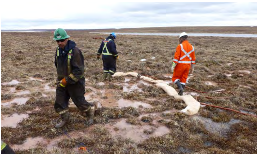
Photograph 3.4-6: Installation of Filter Socks and Sump Pump June 17, 2015
