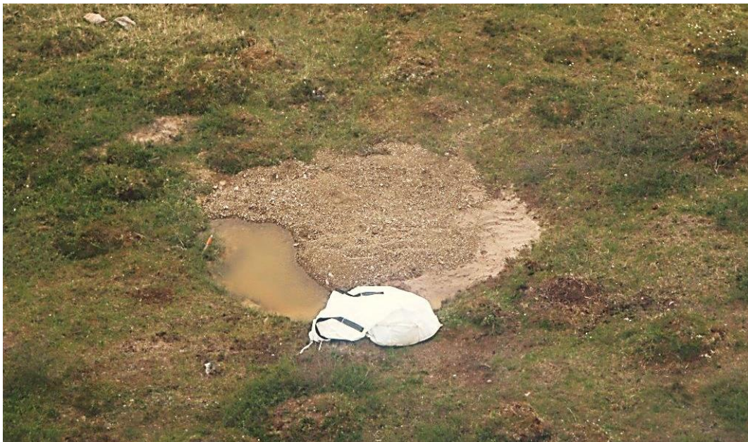
Photograph 3.7-4: Filling Sink Hole at EE-05
