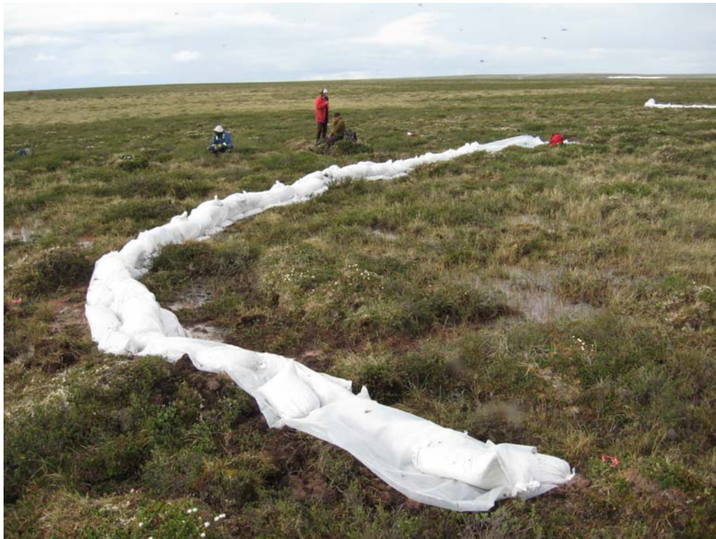
Photo 2 Sandbag berm located along unauthorized release pathway between Andrew Lake and the drill locations.
