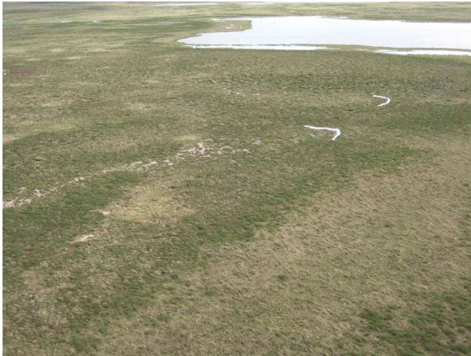
Photo 3 Location of sandbag berms along drainage pathways. Furthest berm is along the unauthorized release pathway where drilling fluids reported to Andrew Lake. The nearest berm was installed along a second pathway and is intended to intercept flow from a second drill.
