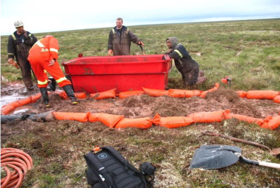
Photo #2: Containment of spill with sand bags
