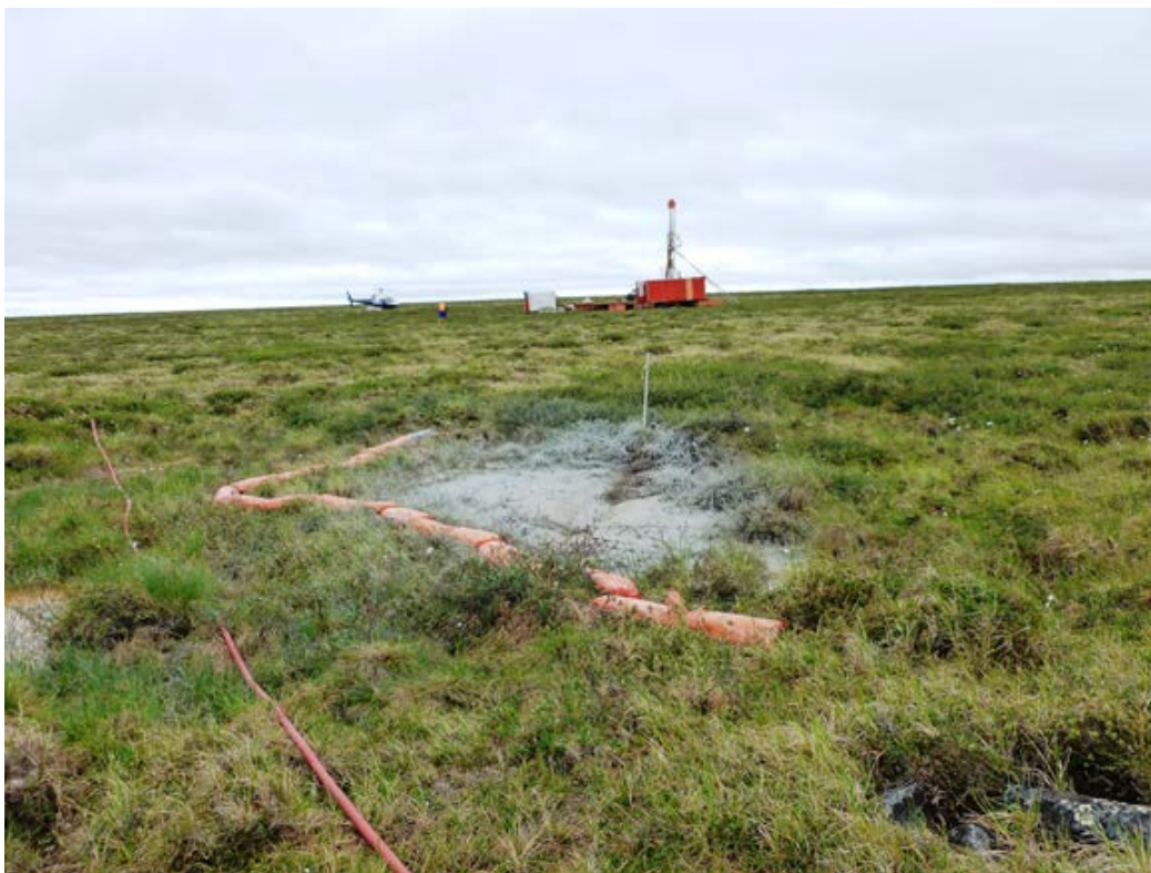
Photograph 5-3 Bermed Cuttings – July 17, 2014
