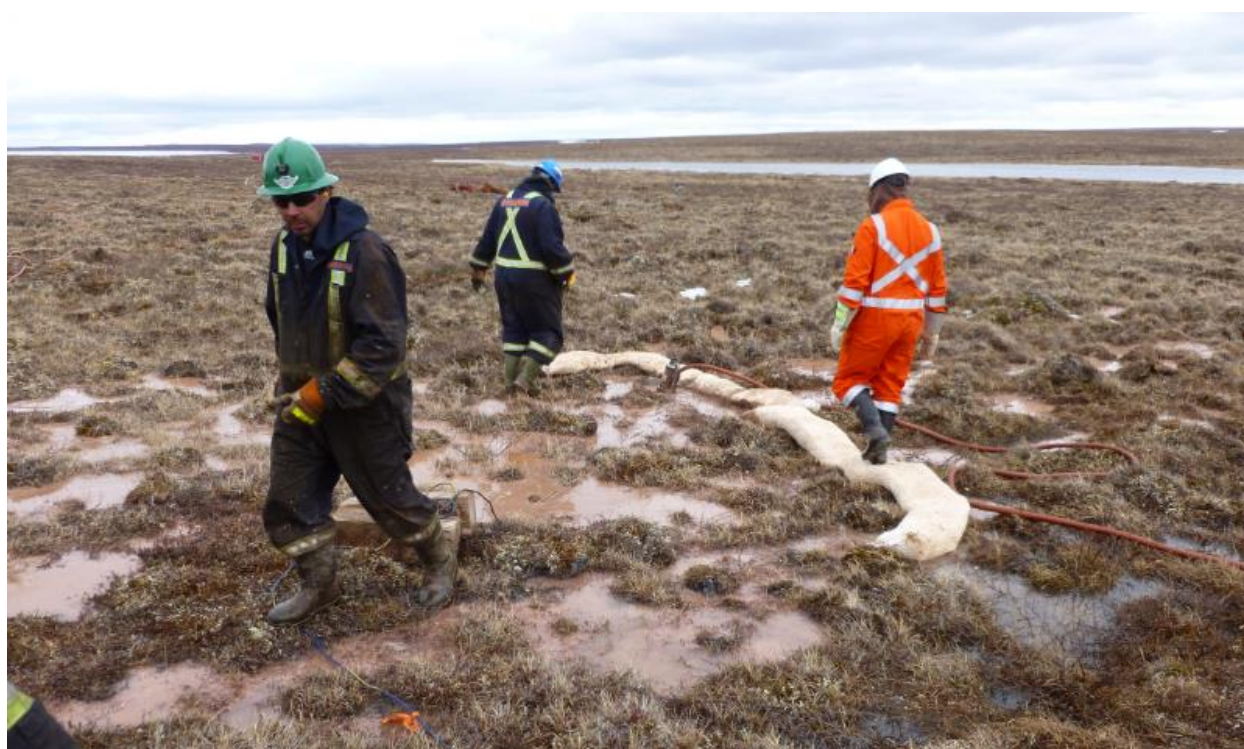
Figure 2. Installation of Filter Socks and Sump Pump on June 17, 2015
