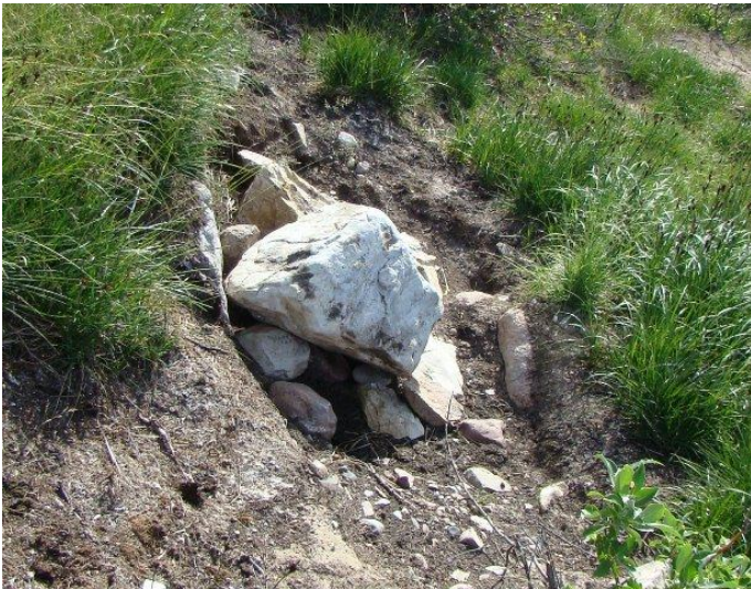
Photographs 4 & 5: Former sump locations were backfilled with large rocks but not restored adequately. Backfill materials are too large for proper contouring and compaction to prevent permafrost degradation.
