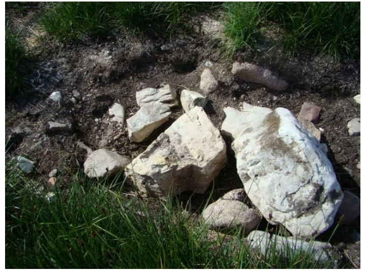
Photographs 4 & 5: Former sump locations were backfilled with large rocks but not restored adequately. Backfill materials are too large for proper contouring and compaction to prevent permafrost degradation.
