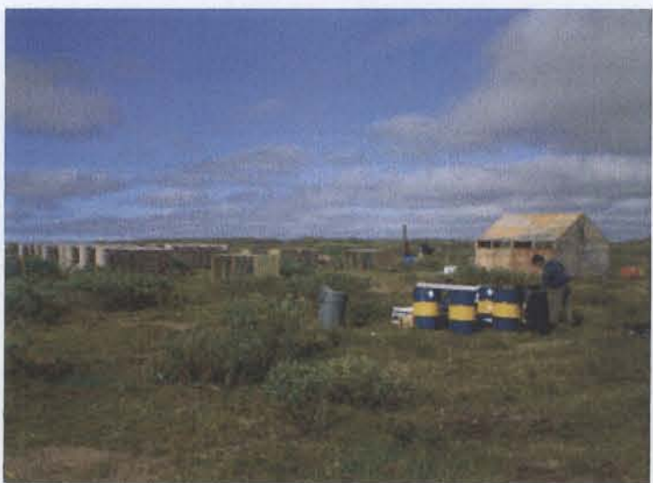
Photo 15. Partial drums of fuel being consolidated for flying. The core logging tent frame is removed and the core shack is undergoing demolition.
