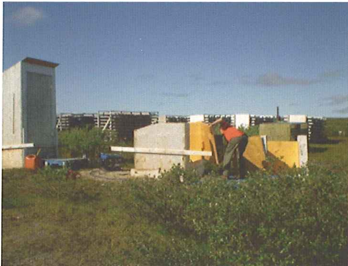
Photo 17. First outhouse being demolished at Kirwan Camp.
