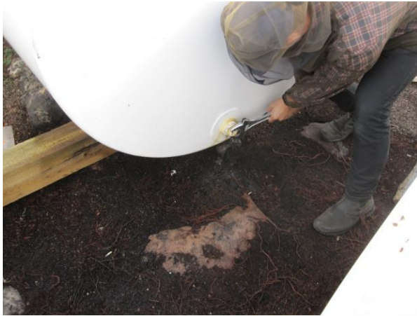
Figure 26: #15-379 – Bulk tank #8 Leak repair
