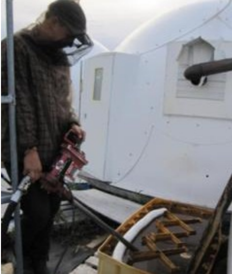
Figure 18: Emptying of secondary containment.
