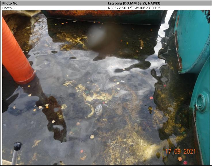
Sheen on the water in the secondary containment berm
