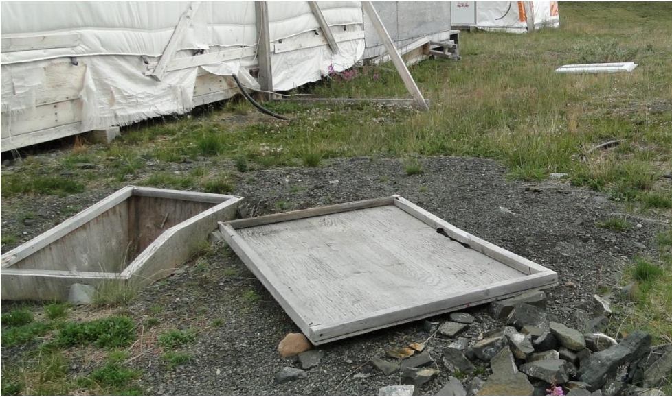
Figure 10. Pit presents a general hazard. We put the lid on and weighted it down.
