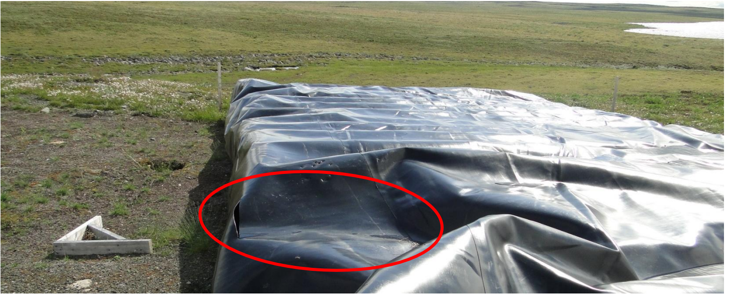
Figure 7. Berm 2 - gash evident in the top, on up-slope side. Water has pooled at that point, so there is likely water in the berm.
