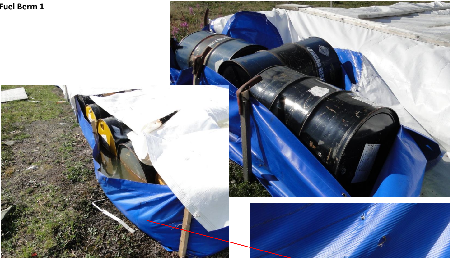
Figure 5. Berm 1 full of water on down-slope side. Puncture hole in side is weeping contaminated water (shown beside).
