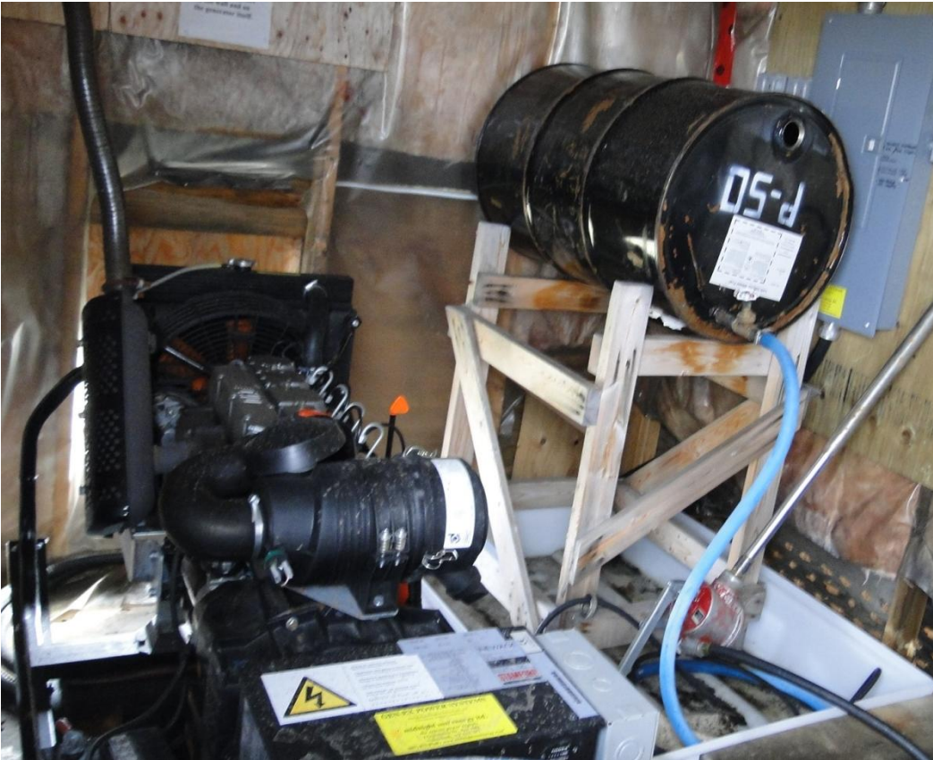
Figure 11. Barrel with no cap, and hose attached. While this barrel is currently in containment, it could be knocked over by wildlife and has no cap on it. I could not get in to the shack far enough to test whether it was full.
