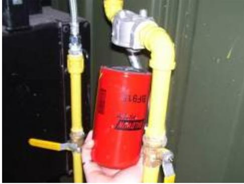
3. Before installing the filter lubricate the seal on the new filter.
