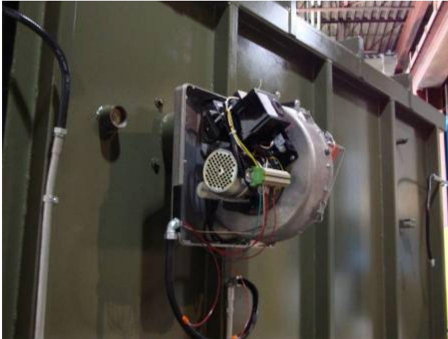
**NOTE** Burner is shown without cover installed.
