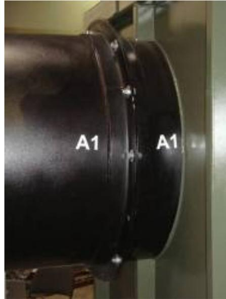
Correctly Installed Breech on Primary Chamber
