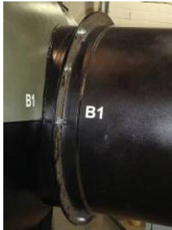
**Correctly installed Breech on Secondary Chamber**
