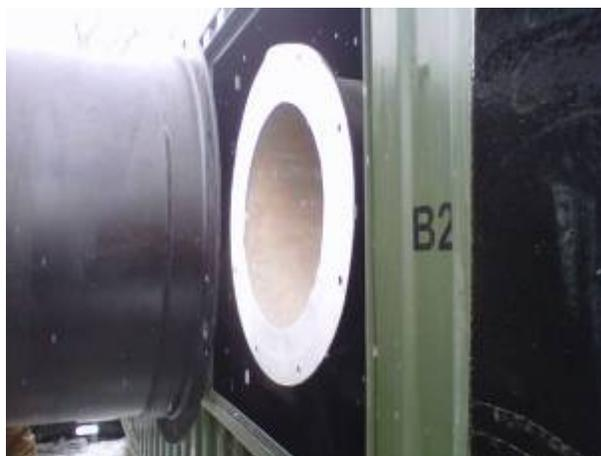
**Correctly Installed Gasket**
