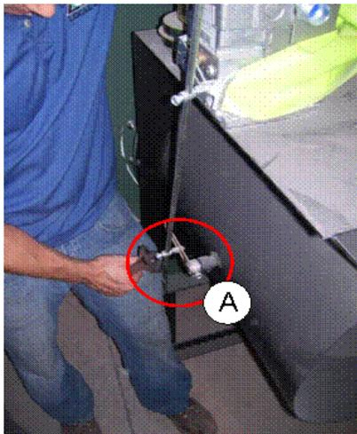
A. Damper Crank arm and connection to Damper and Rod
