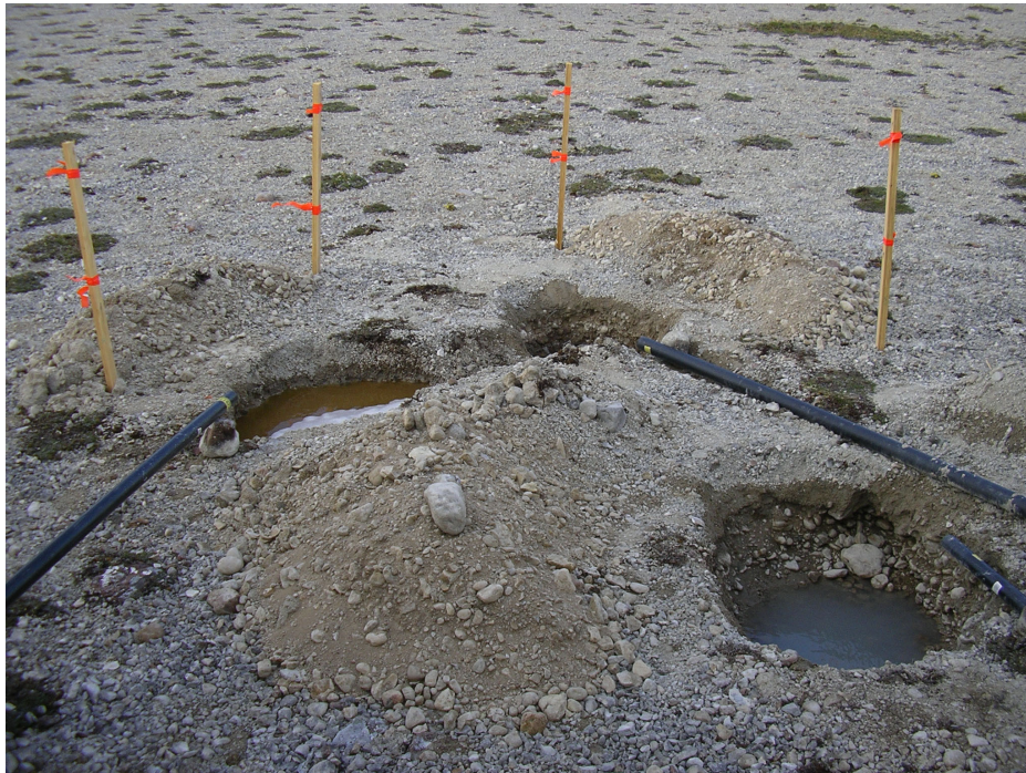
The 3 Greywater Sumps During Use
