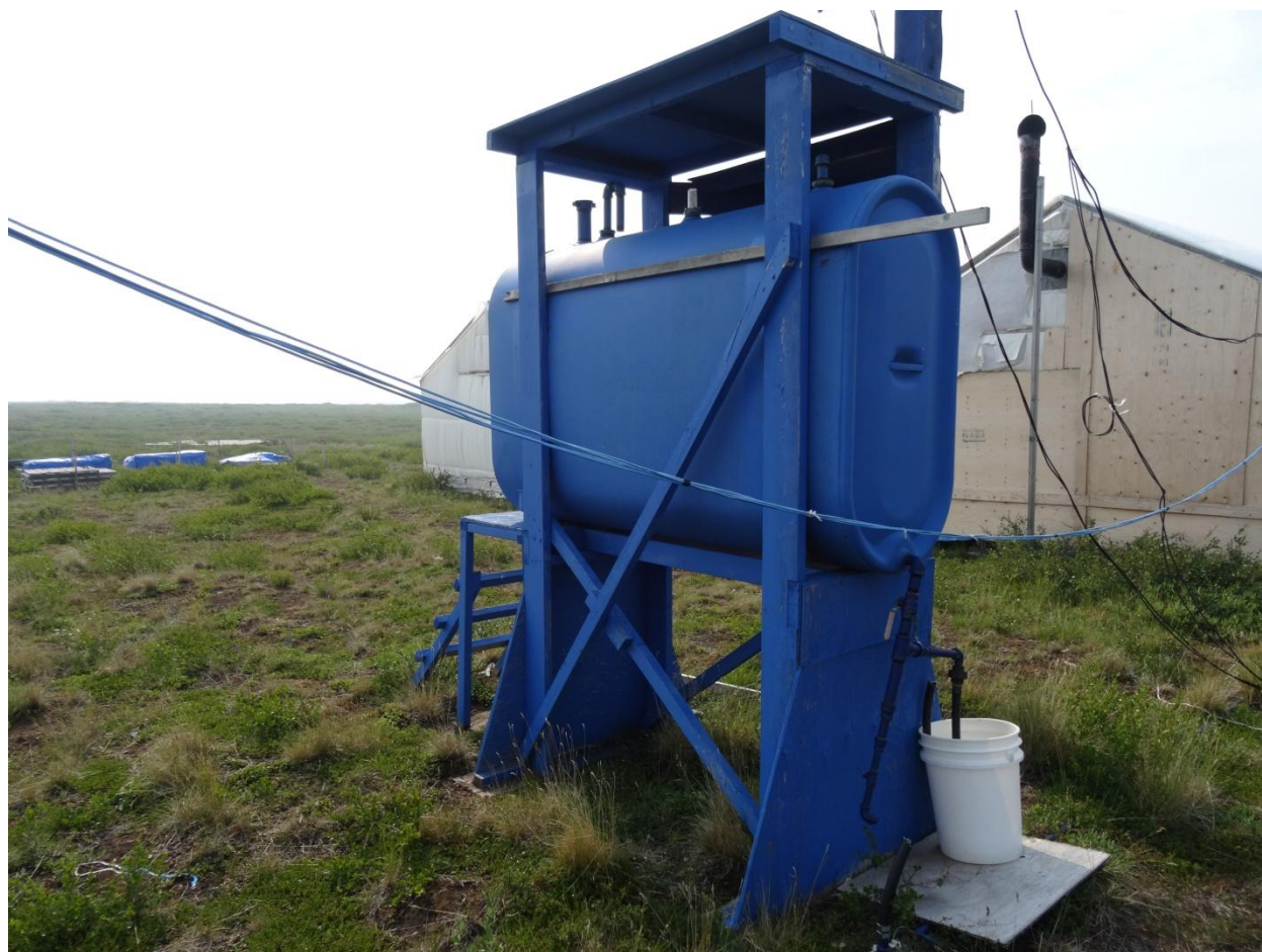
Figure 11. Tall heating fuel setup. No secondary containment for the tank and valves.
