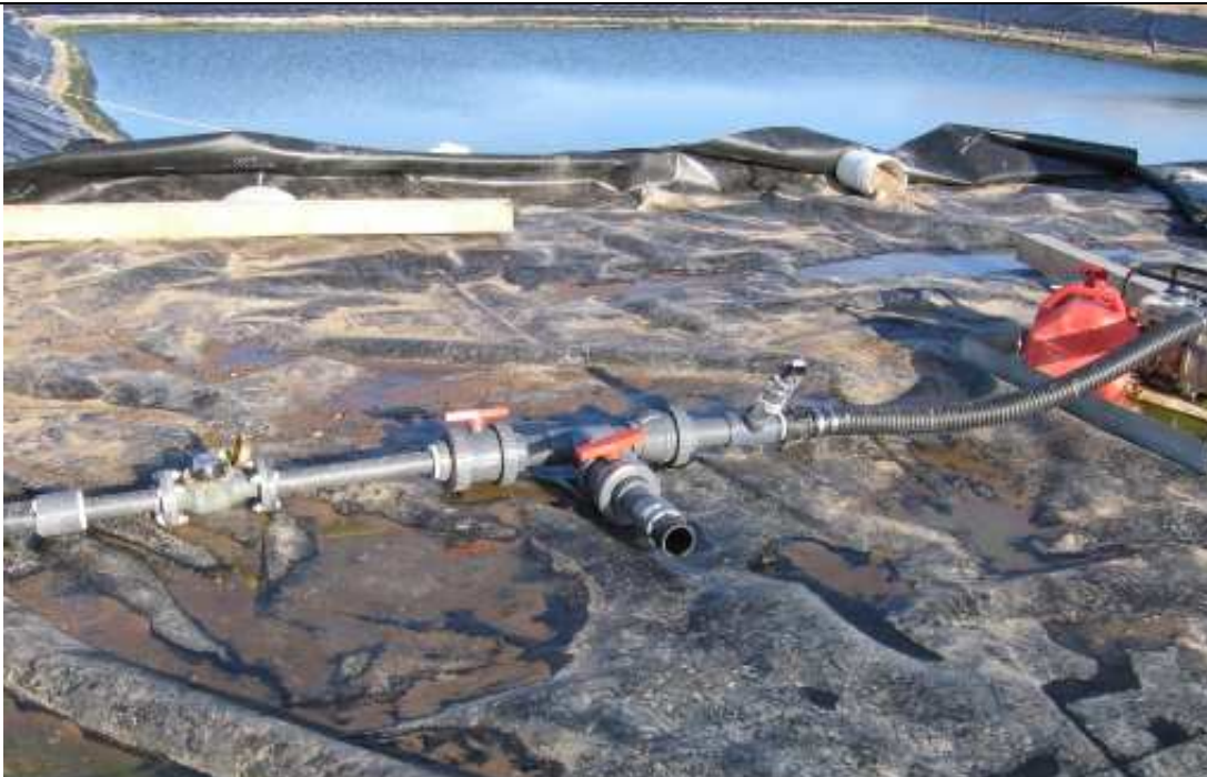
Photograph 1 Treatment System Influent Pump and Flowmeter
