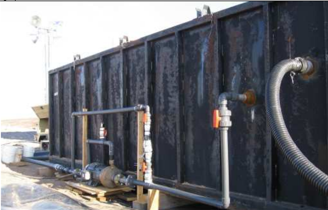
Photograph 4 Dissolved Air Floatation Pump
