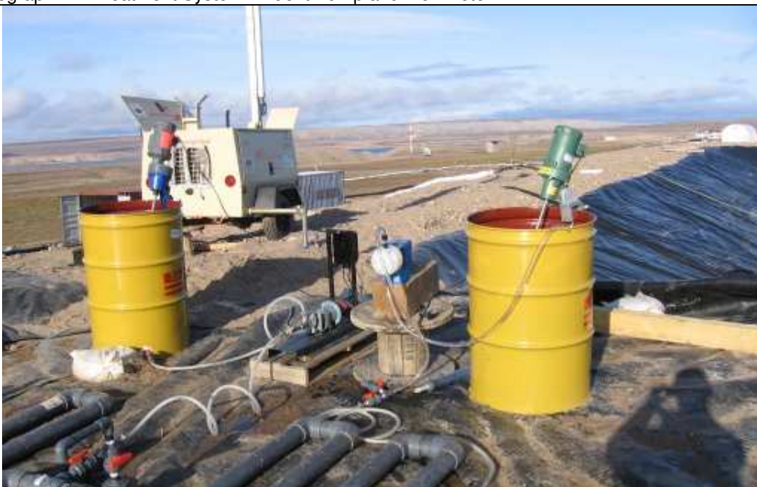
Photograph 2 Aluminum Sulphate and Polymer Dosing Systems with Flocculation Piping
