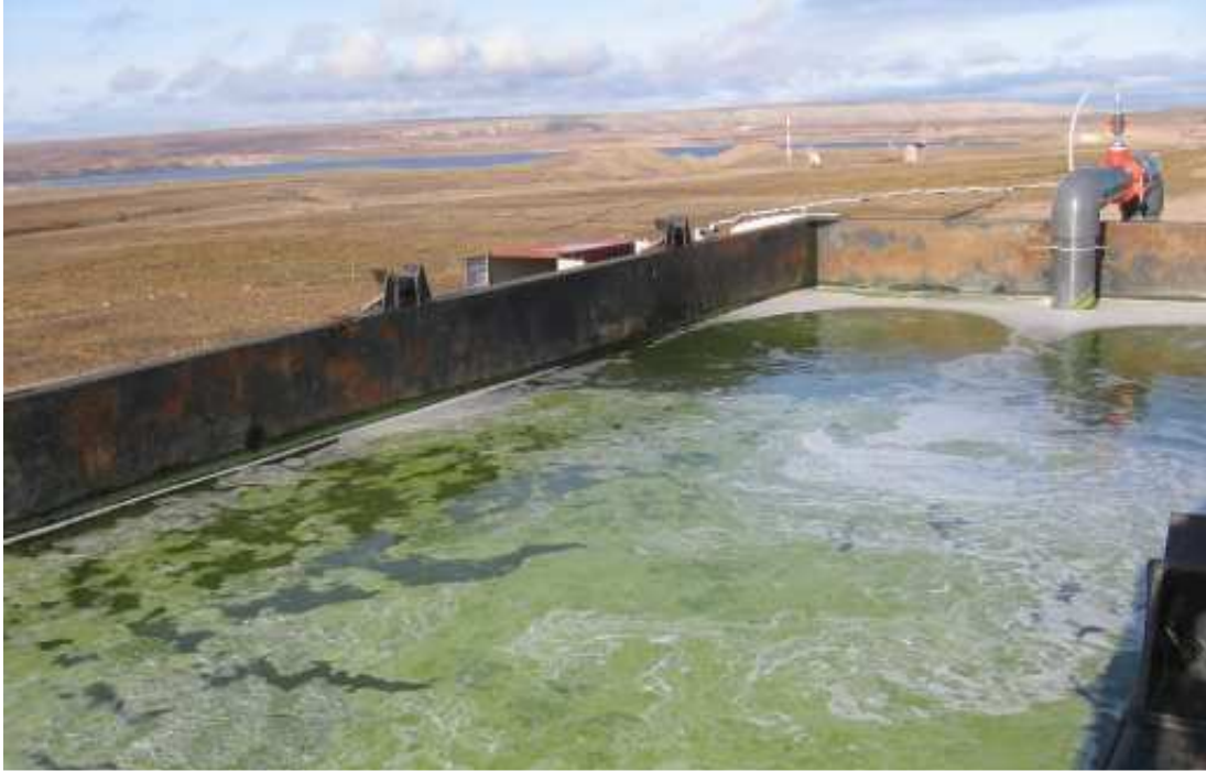
Photograph 3 Dissolved Air Floatation Tank
