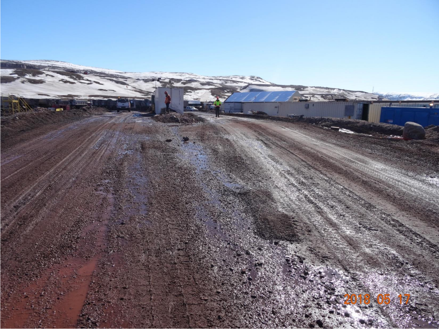
Figure 12: contact water exiting fuel station module
