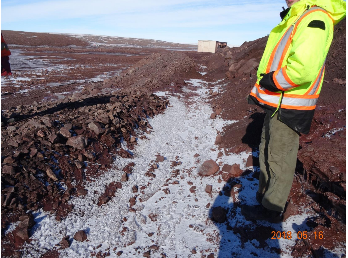
Figure 3: erosion or incompleteness of ditch wall seen in the center of the photograph location near the “Ehouse”
