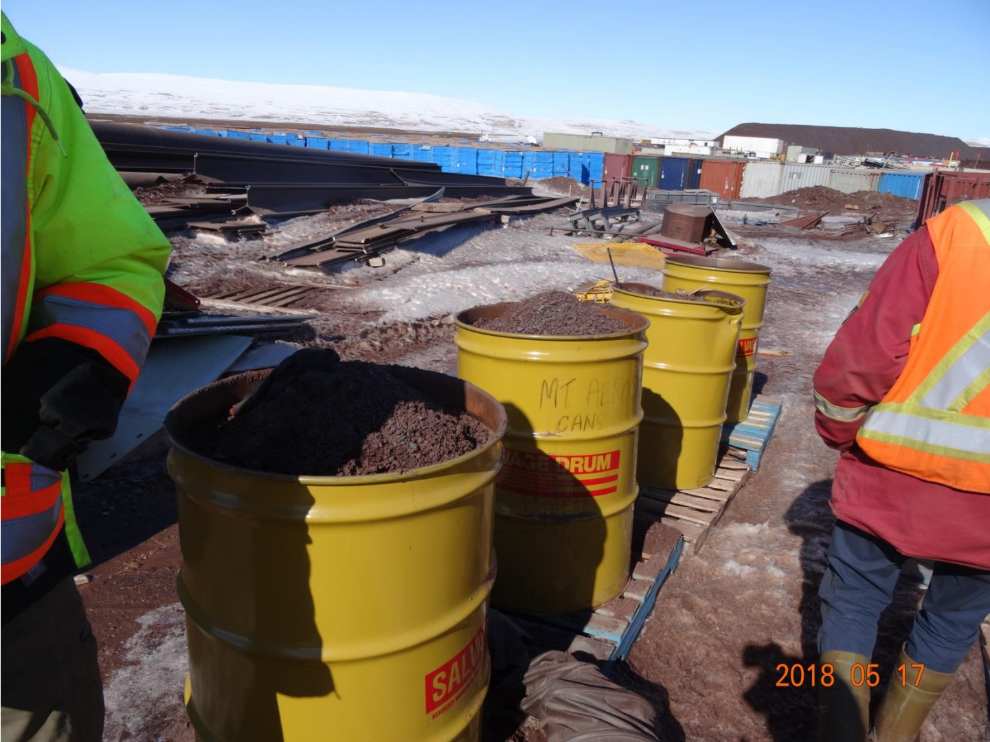
Figure 11: contaminated soil in unsealed containers near batch plant
