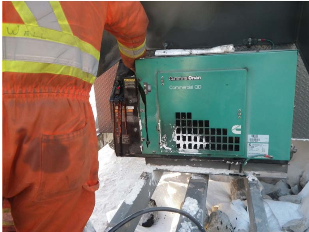
Photo 1 - Spill location- Oil dripping from the unit (left)
