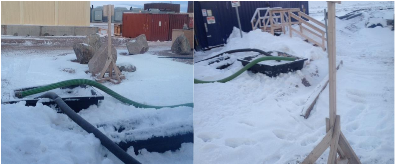
PHOTO 2/3 – Discharge Pipe Spill Clean-up and Berm Extension/Barricade
