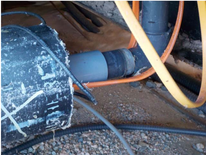
Photo 1 – Failed Joint
