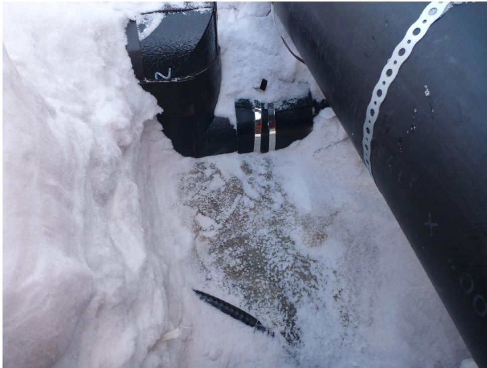
Photo 2 – Frozen sewage encasing half of the discharge pipe
