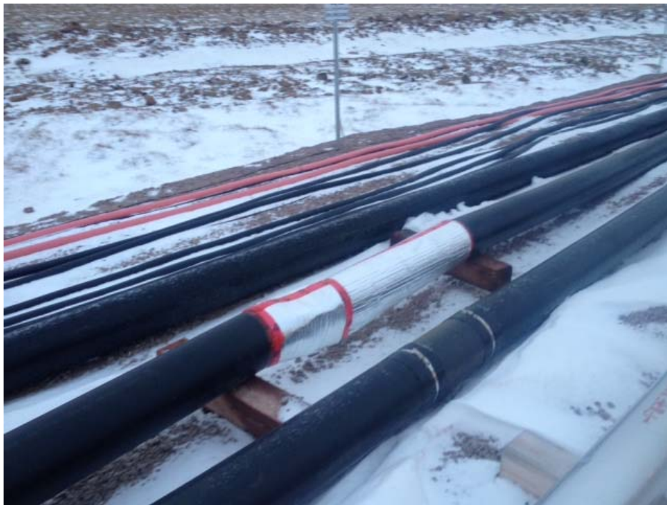
Photo 2 – Repaired Joint
