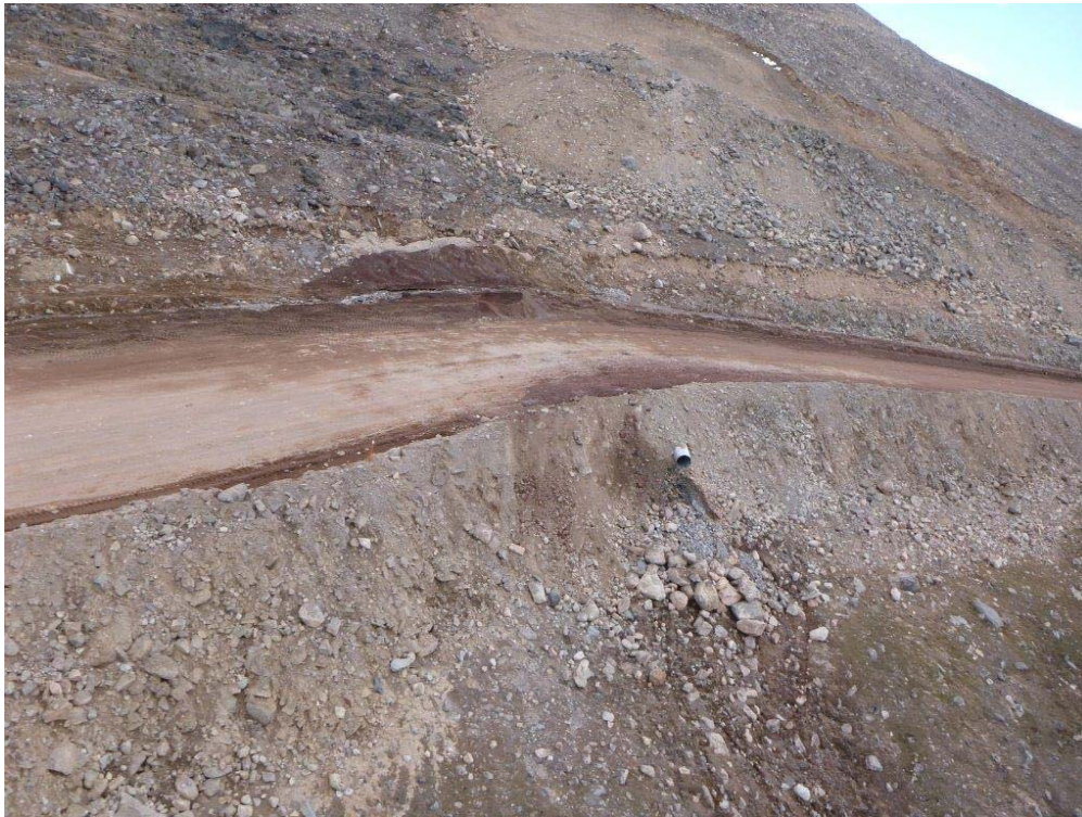
Photo 1: Culvert at Km 107 of Mine Haul Road. Sediment released downstream from this location on June 26 and 27 from erosion of road embankment and upstream ditches.
