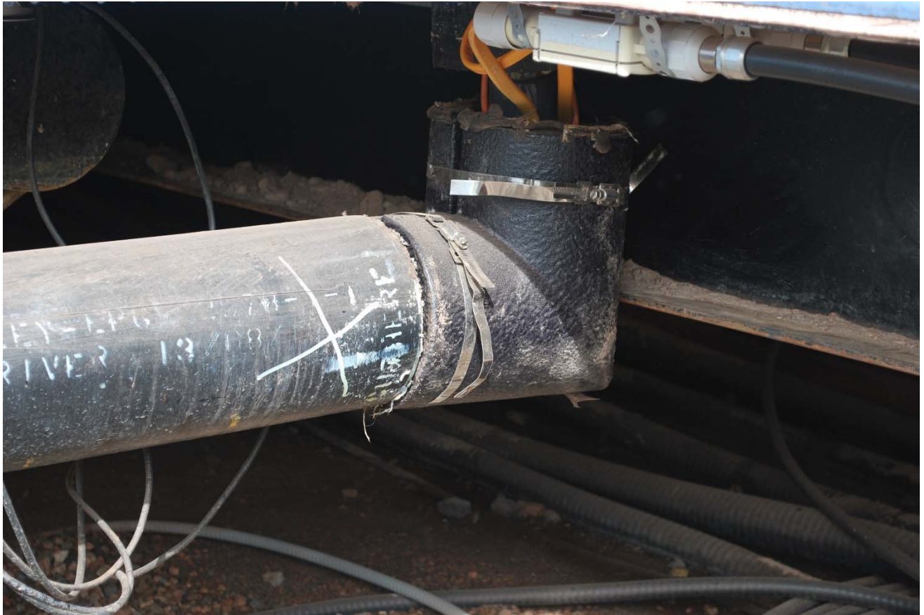
Photo 3 – Repaired Joint
