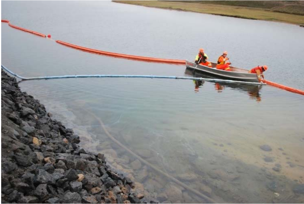
Photo 1 – Spill Response – Capturing Sheen with Booms
