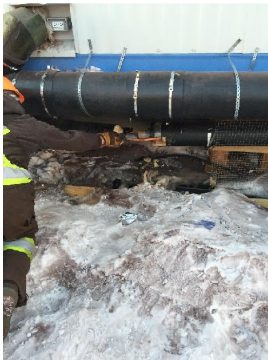
Photo 2 – Discharge Pipe Being Repaired
