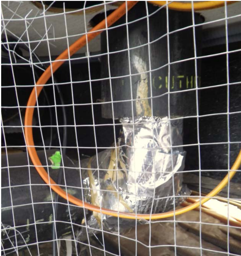
Photo 3 – Repaired Joint
