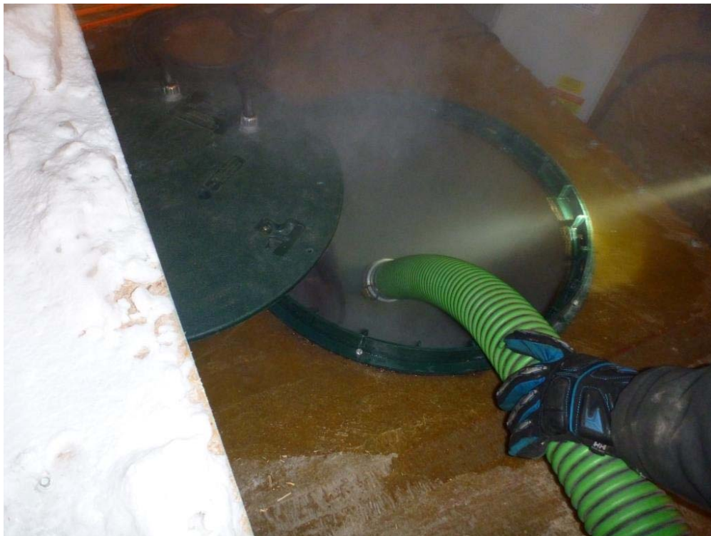
Photo 2 – Pumping out the lift station by vacuum truck
