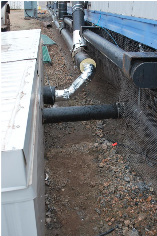
Photo 3 – Repaired Joint
