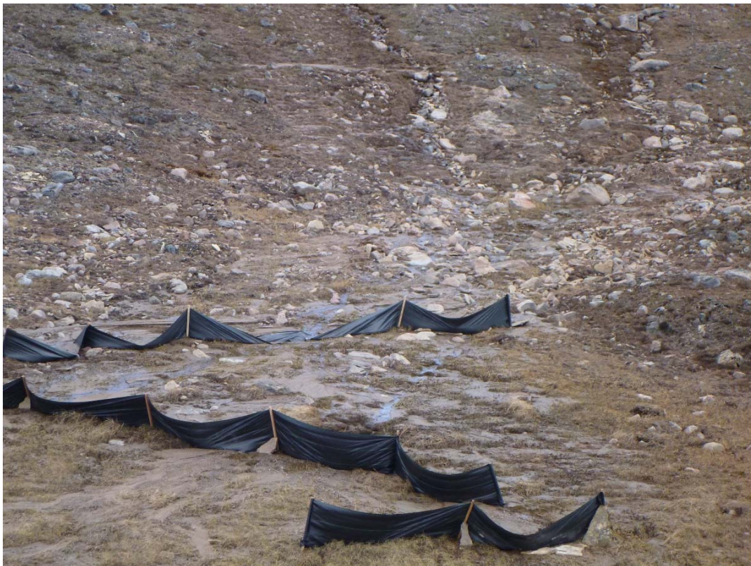
Photo 4: Silt fences effectively trapping sediment release downstream of Culvert at Km 107 on June 27.
