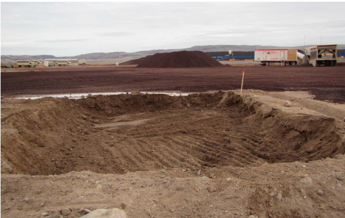
Photo B.5: West Generator Footprint after Excavation
