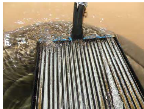
Uneven aeration in membrane tank
