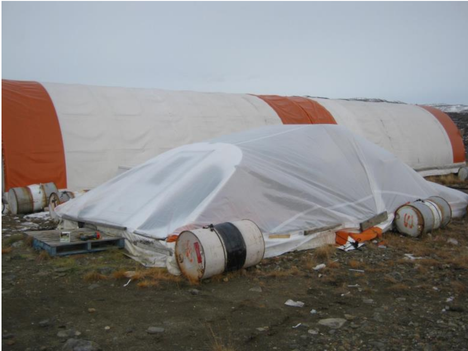
Figure 24 – Damaged hut covered with tarp
