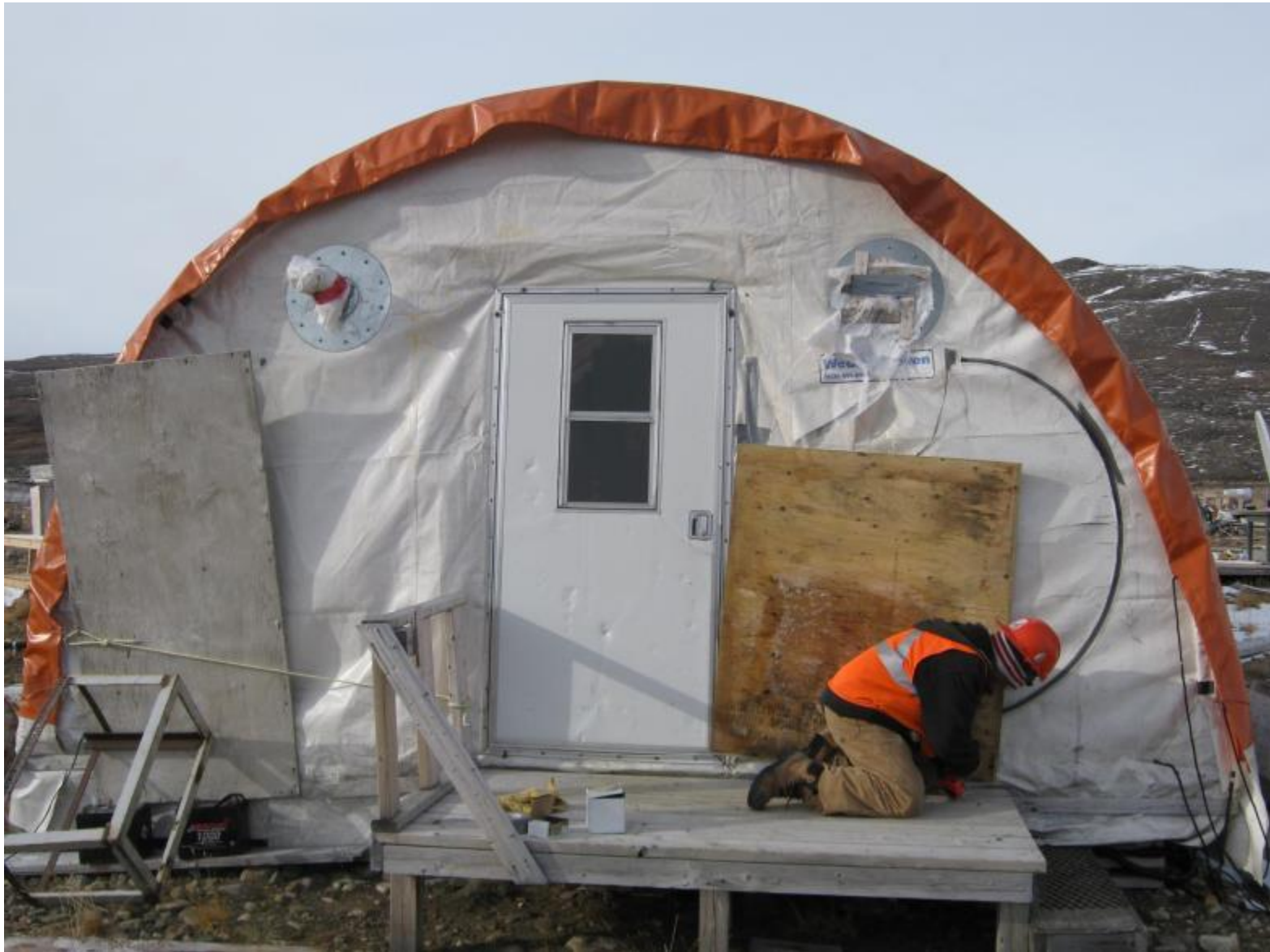
Figure 32 – Boarded up hut openings
