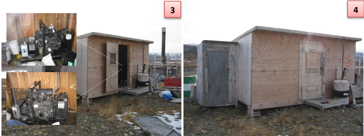
Figures (3) and (4) – Securing the shack housing the generators
