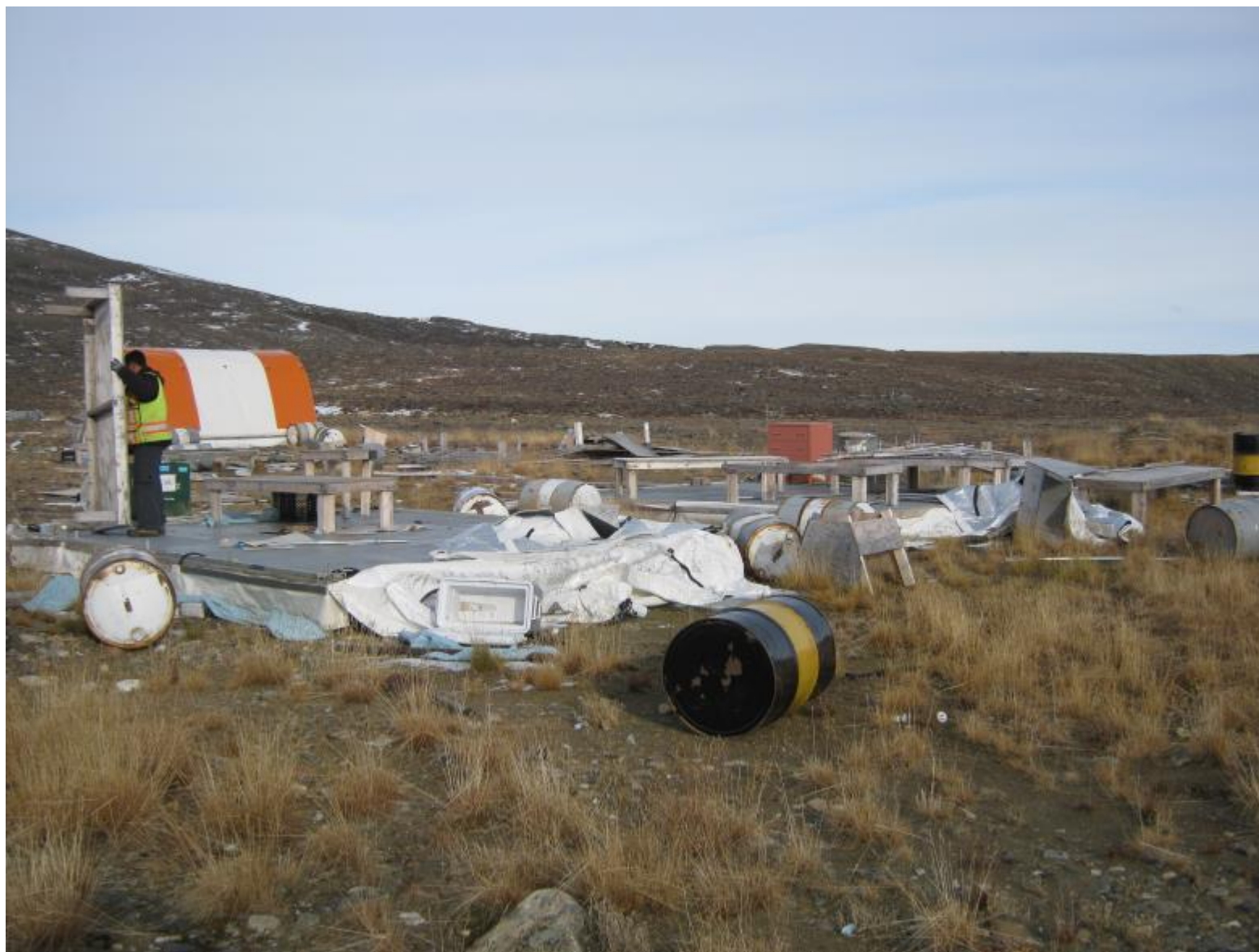
Figure 11 – Salvaging wood for repairs; general site view
