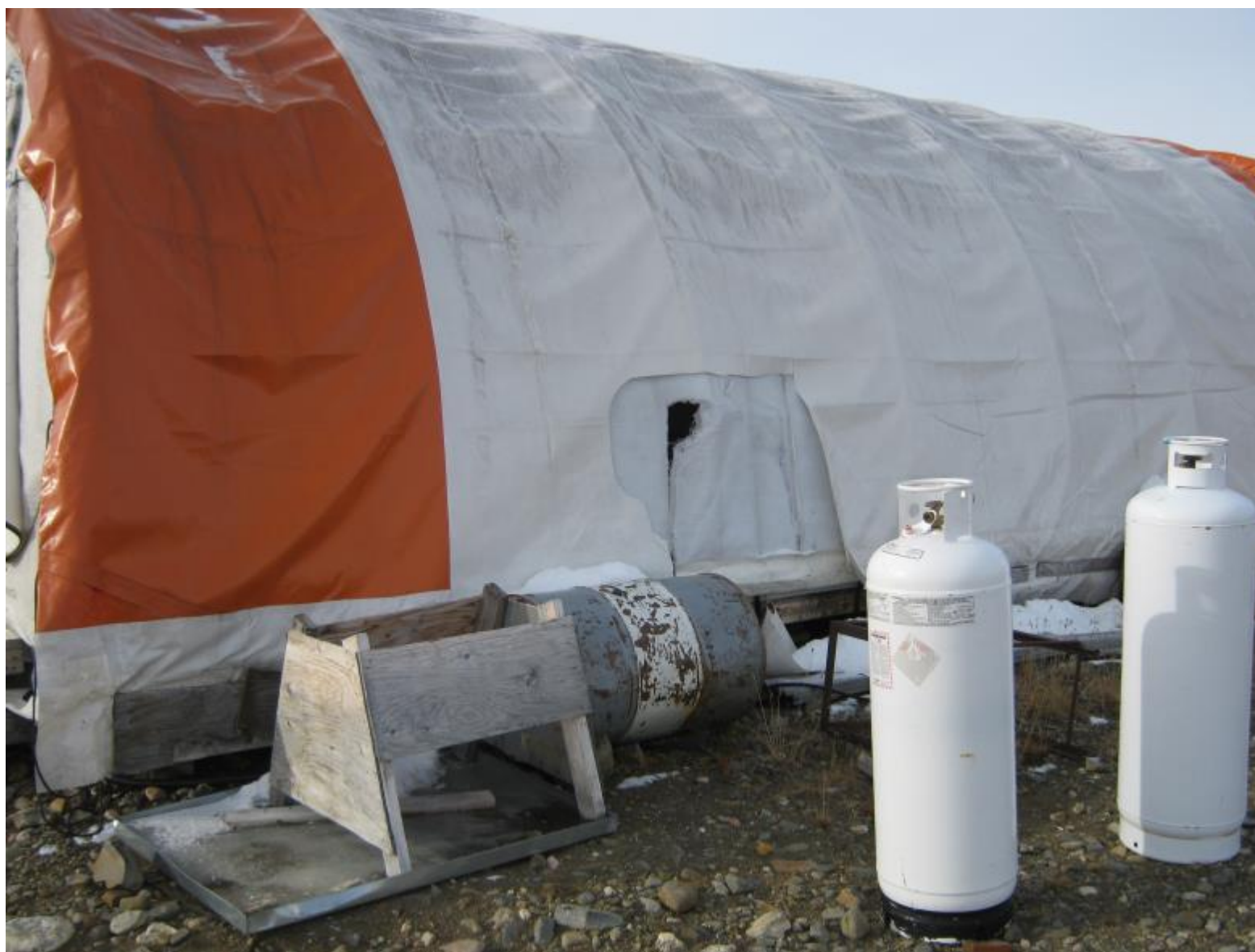
Figure 14 – Torn tent on hut
