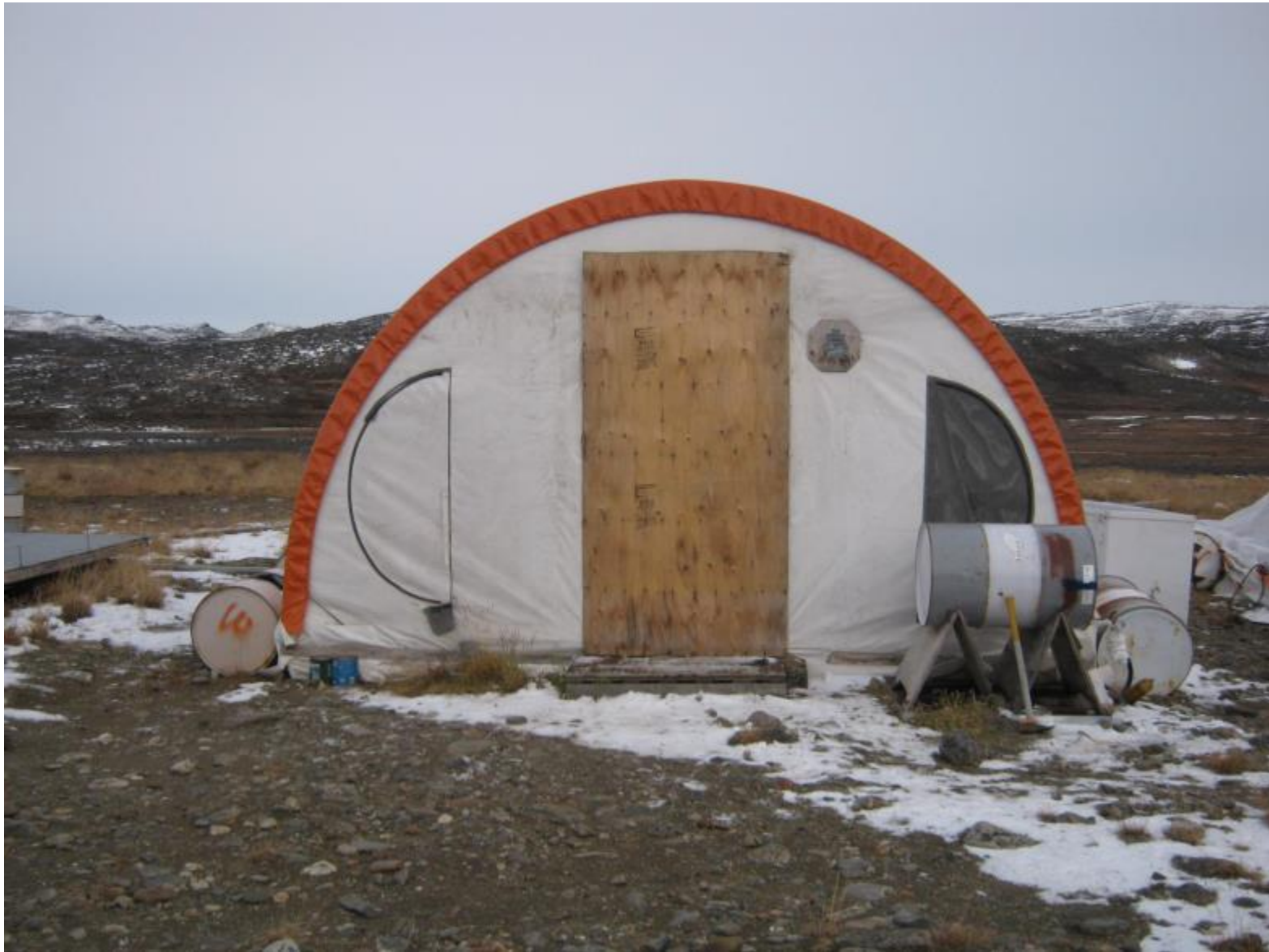
Figure 22 – Boarded up hut
