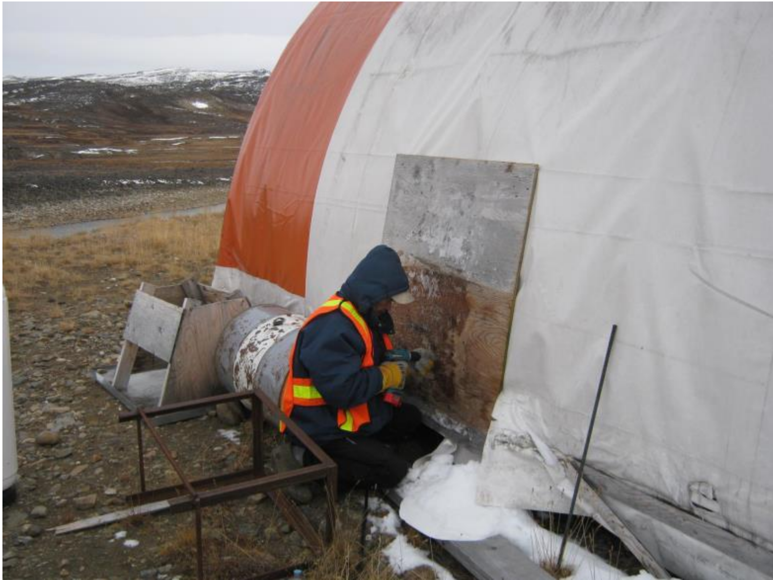
Figure 23 – Boarding up torn tent section on hut
