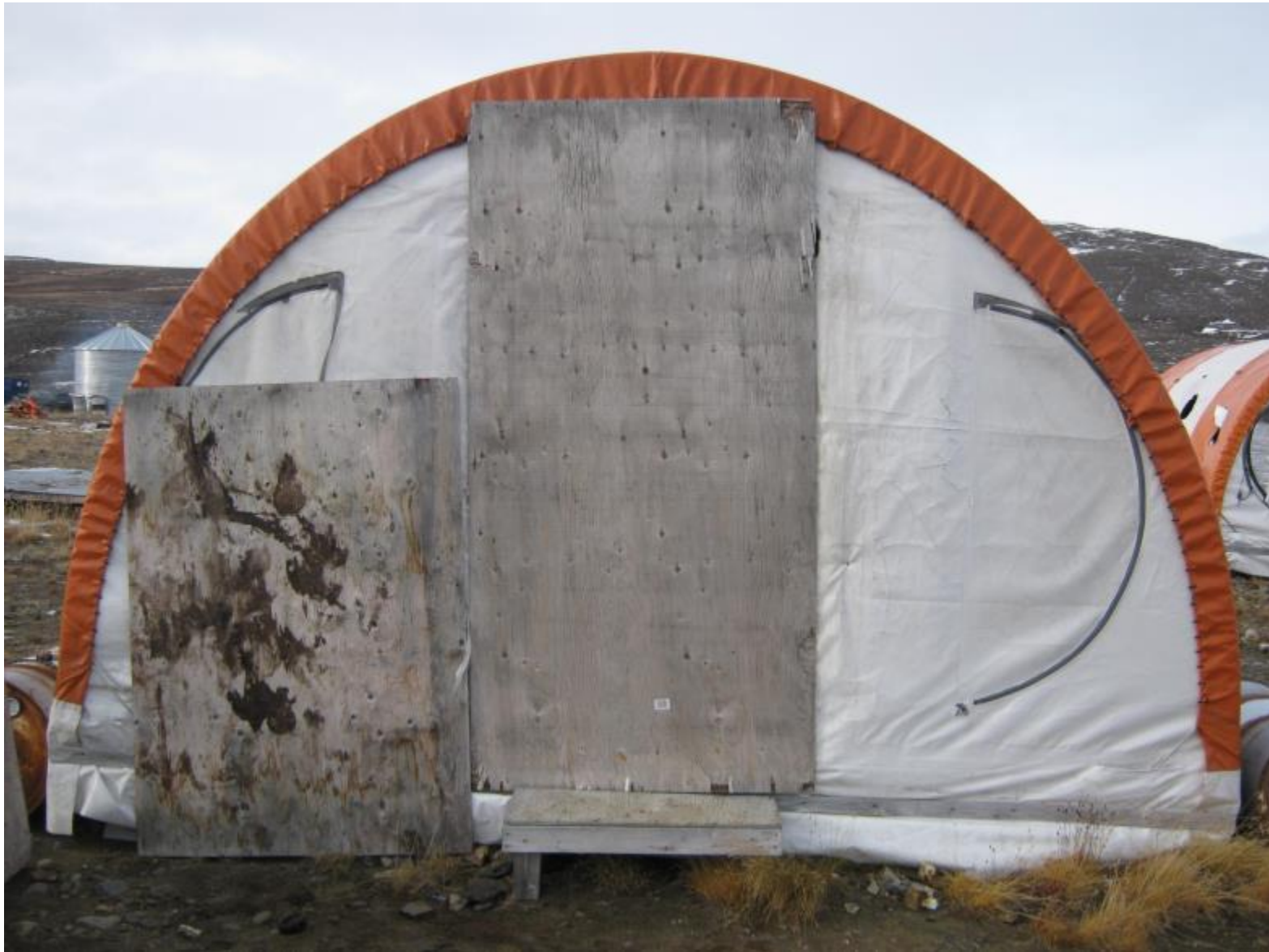
Figure 31 – Boarded up hut openings
