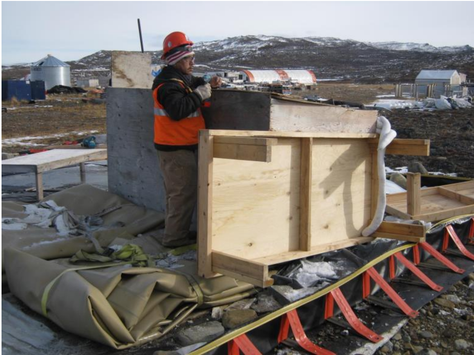
Figure 21 – Boarding up water and fuel pump system
