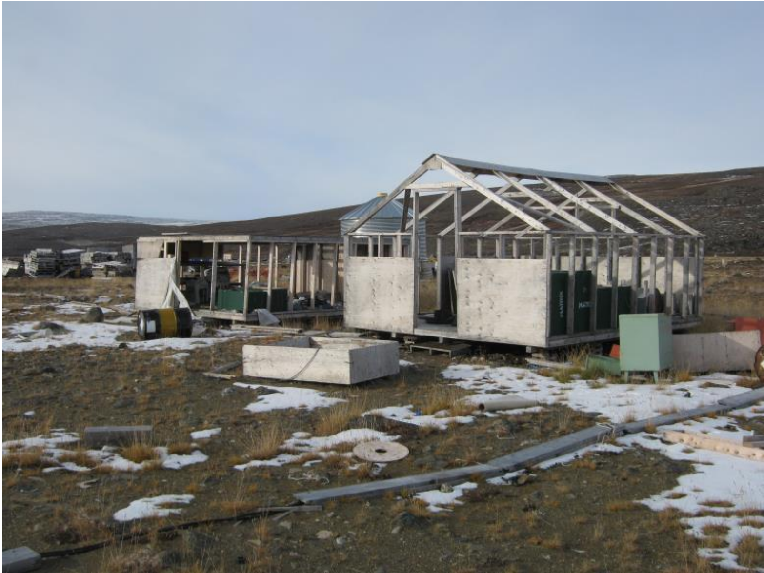
Figure 8 – Camp structures and general site view
