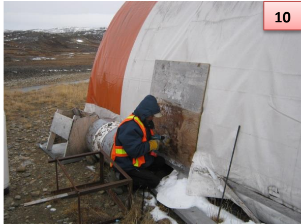
Figures (9) and (10) – Boarding up kitchen/dining hut torn tent sections (side)
