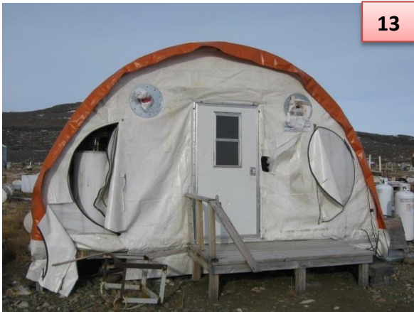
Figures (13) and (14) – Boarding up kitchen/dining hut torn tent sections (front)
