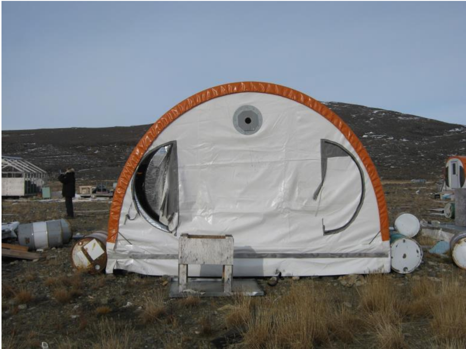
Figure 12 – Ripped tent opening on hut
