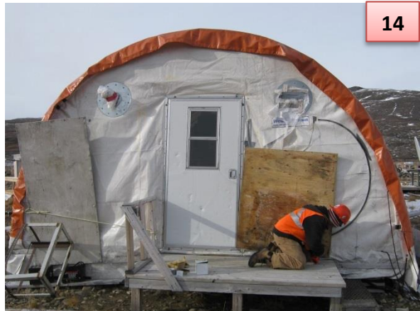
Figures (13) and (14) – Boarding up kitchen/dining hut torn tent sections (front)
