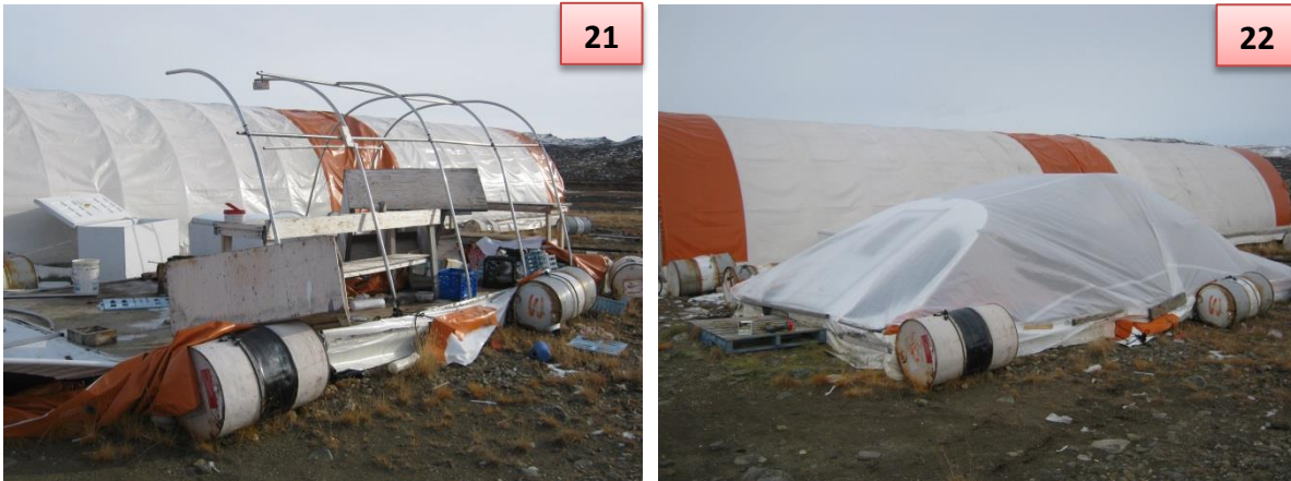
Figures (21) and (22) – Securing damaged hut
