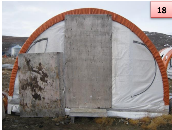
Figures (17) and (18) – Boarding up openings and tears on tent
