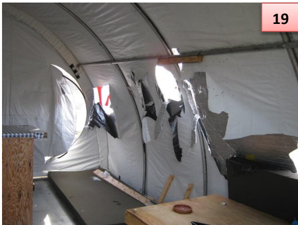
Figures (19) and (20) – Covering tears on tent (view from interior/ exterior)
