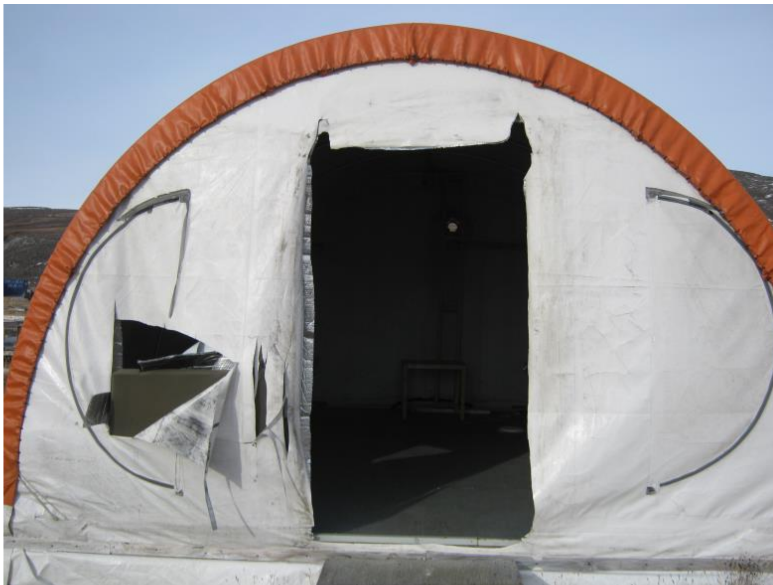
Figure 13 Torn tent and detached door on hut
