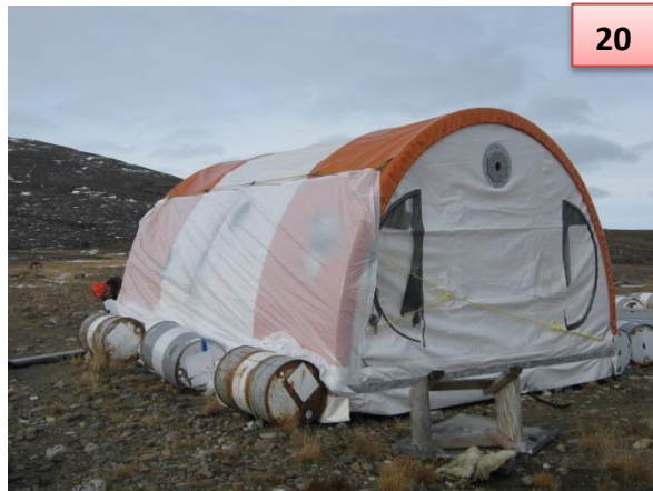
Figures (19) and (20) – Covering tears on tent (view from interior/ exterior)
