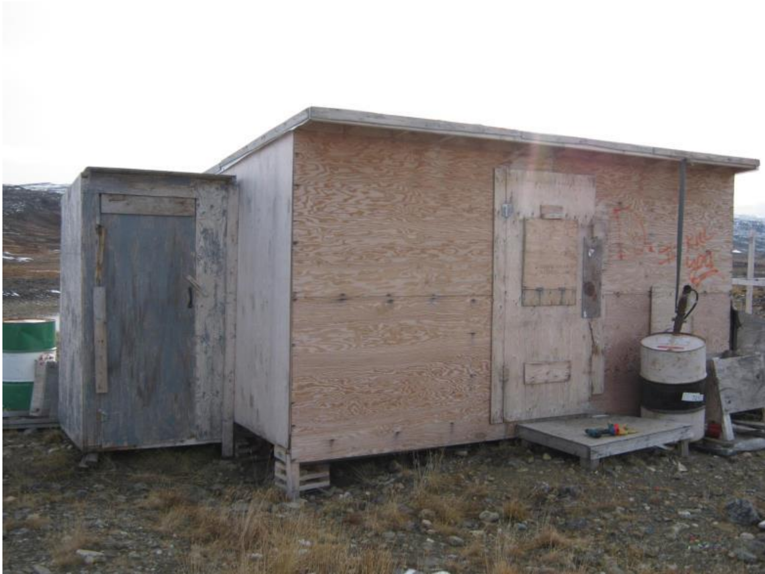
Figure 34 – Shed and attachment doors reinstalled and shut
