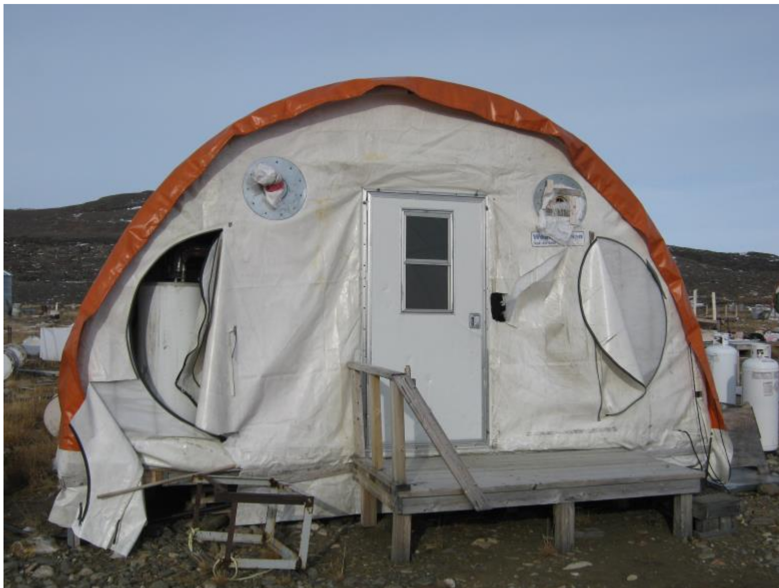
Figure 15 – Torn tent sections on hut
