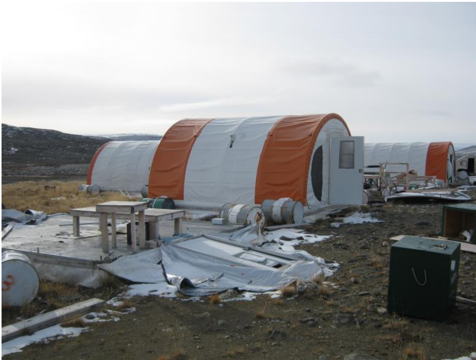
Figure 6 – Damaged huts; general site view
