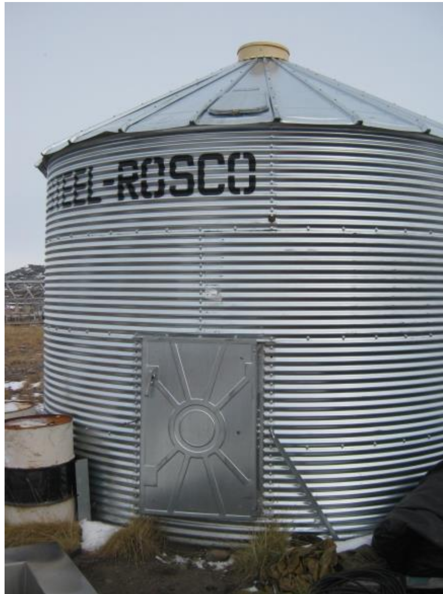
Figure 25 – Door and roof hatch repaired and properly shut
