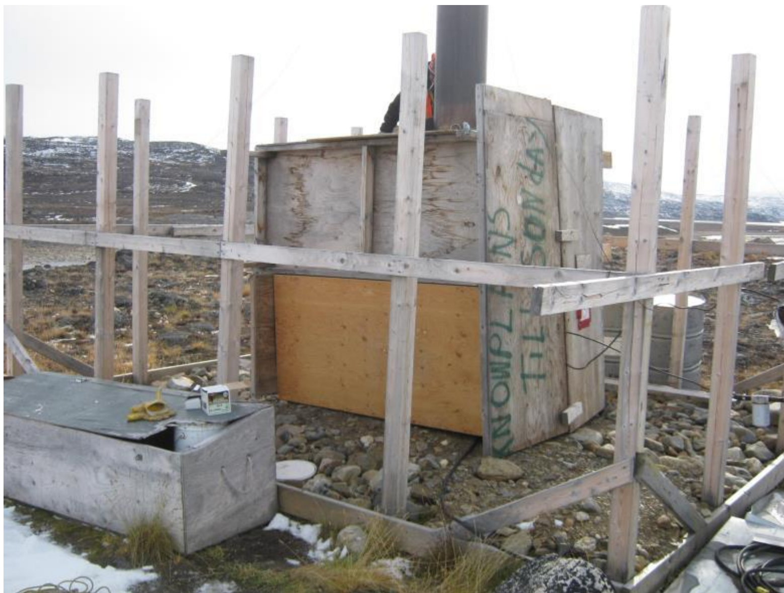
Figure 33 – Boarding up incinerator
