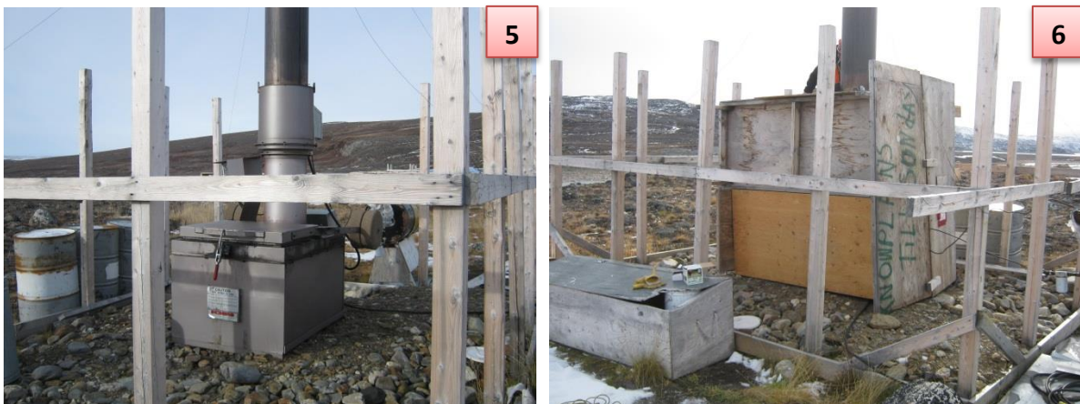
Figures (5) and (6) – Protection box around the incinerator
