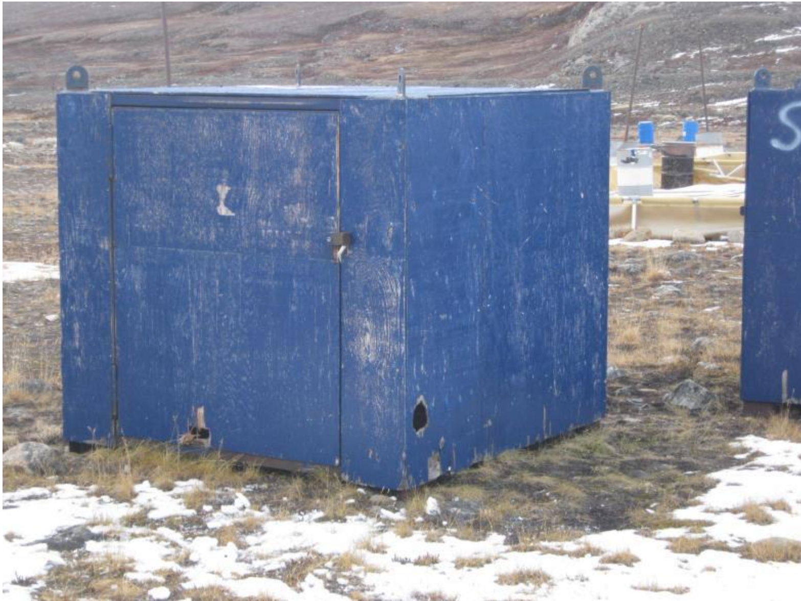
Figure 26 – Repaired (door) shed
