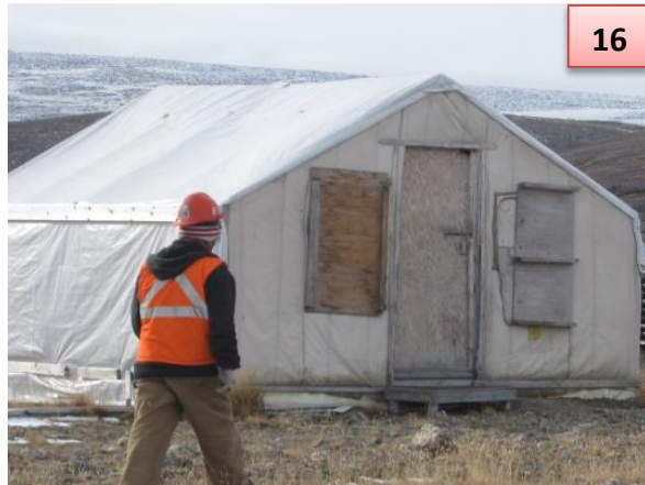
Figures (15) and (16) – Boarding up door and window openings
