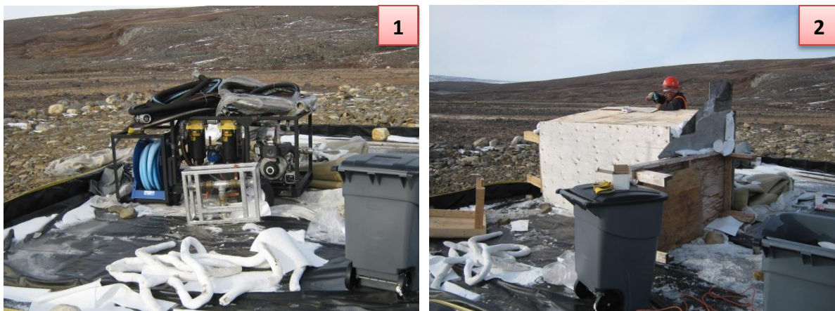
Figures (1) and (2) – Barricading the pumping system
