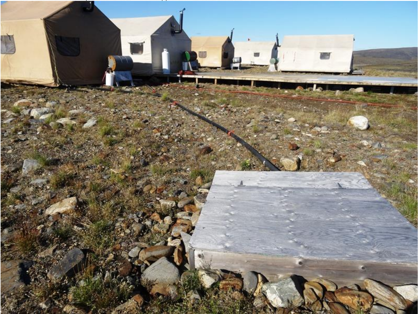
Photo 3: Sump where greywater is discharged.
