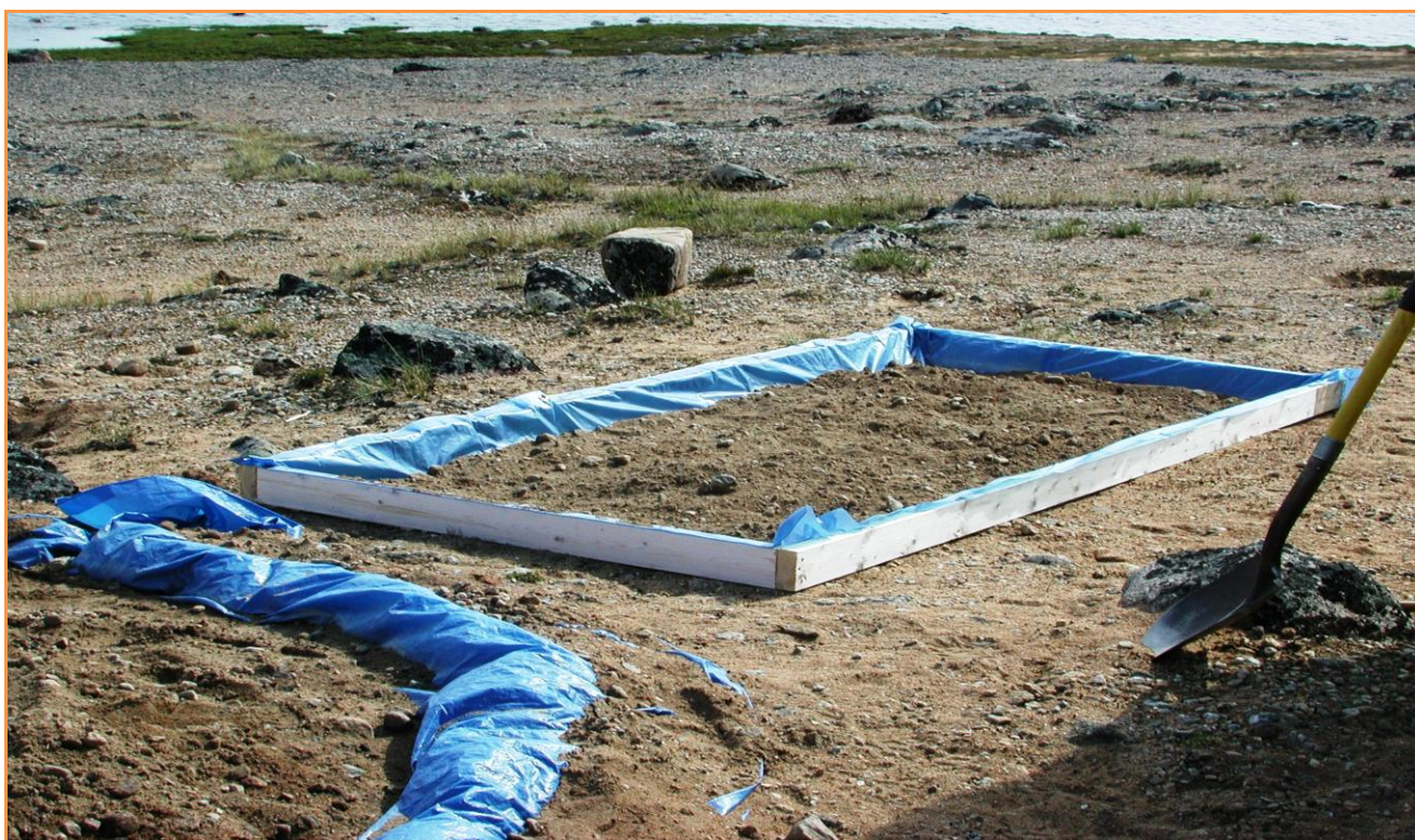
TOP: Camp attendant Hugh Haqpi of Repulse Bay excavates small hydrocarbon spill on 07 July 2009. Refilled petrol drum had leaked over winter from small rupture on its side. ABOVE: Material excavated from diesel spill (when leakage occurred from a faulty bung over winter) was aerating successfully in a wooden box behind camp in late July 2009.
