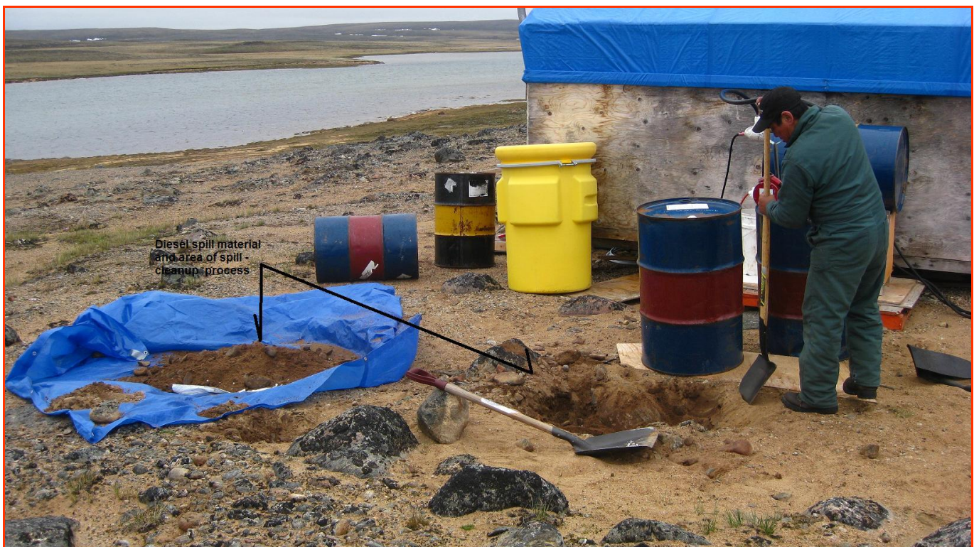
PHOTO 2: CLEANUP IN PROGRESS: DIGGING OUT DIESEL SPILL, NANUQ CAMP, NU
