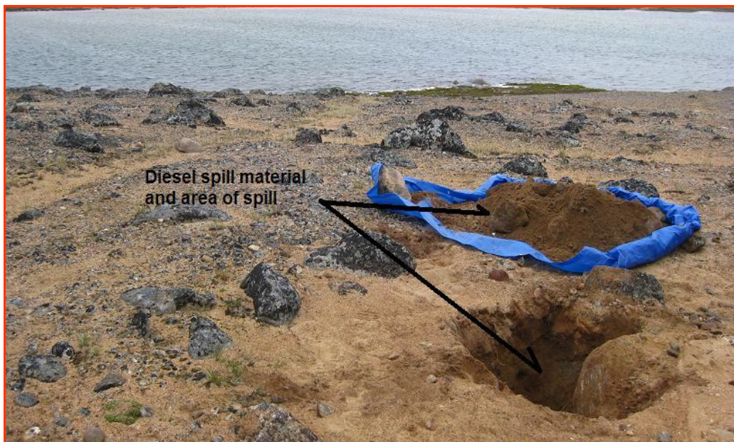
PHOTO 4: DIESEL SPILL MATERIAL TRANSFERRED ONTO TARP, NANUQ CAMP, NU
