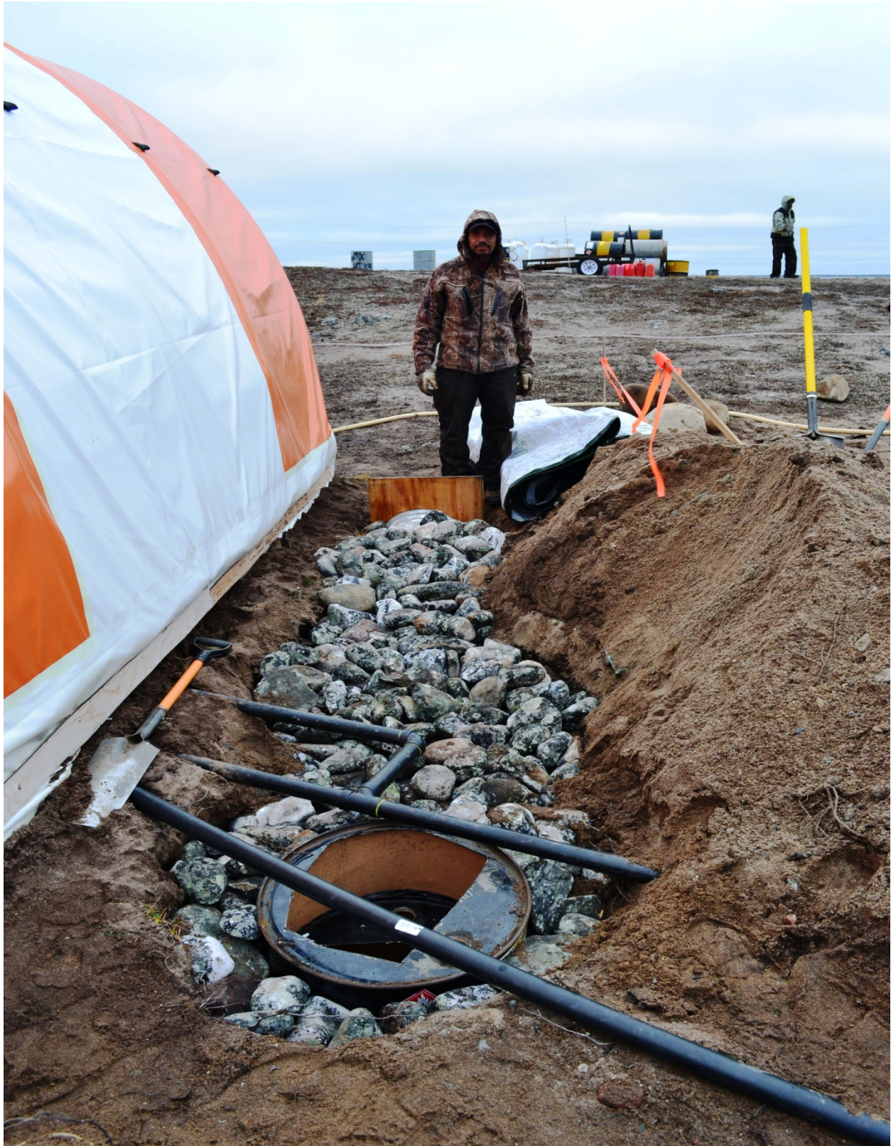
2013 Addition to Camp Grey Water Disposal System
