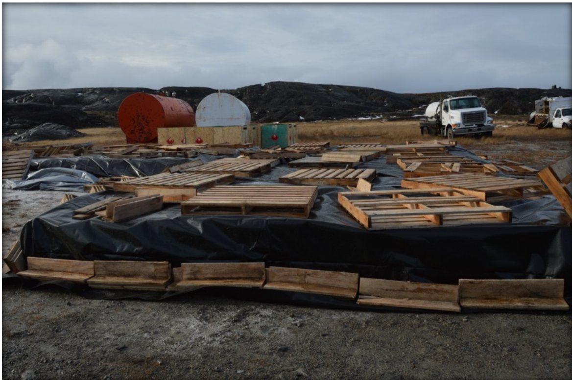
Final winter storage of Jet 1 Fuel in covered berms.
