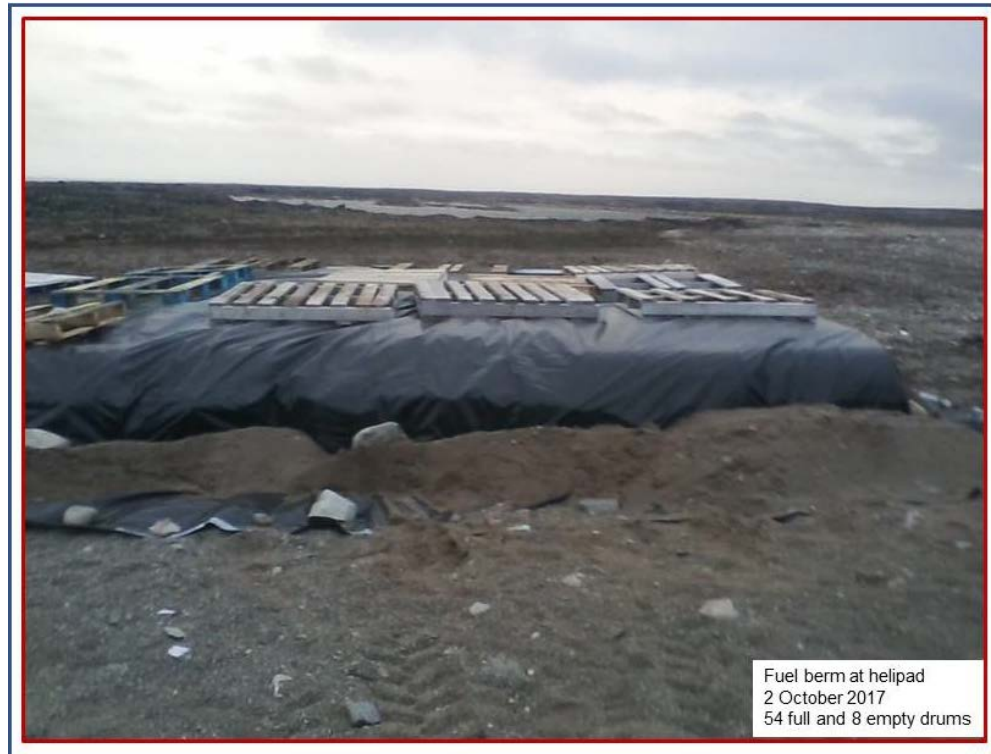
Figure 3. Fuel berm, at the camp heli-pad, with Jet A-1 fuel stored for the winter
