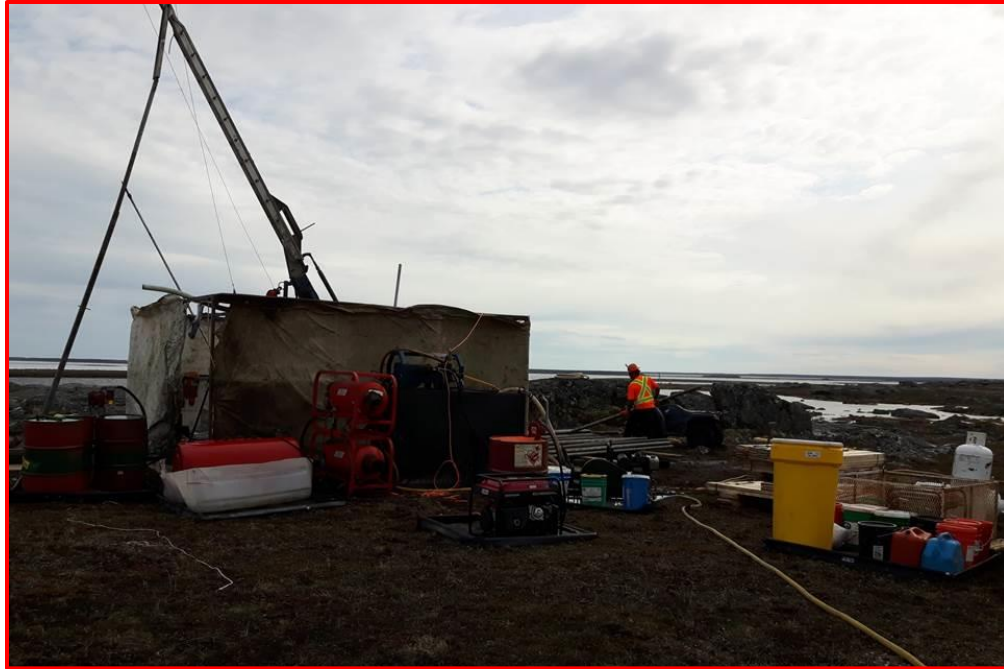
Figure 12. Photo of DDH 19PB075 drilling in progress.
