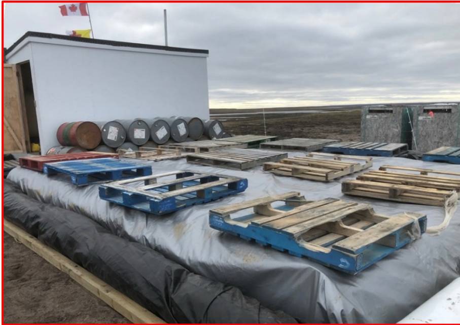
Figure 3. Fuel berm Number 1, at the camp generator shack, with diesel gasoline, waste oil and water heater fuel stored for the winter.
