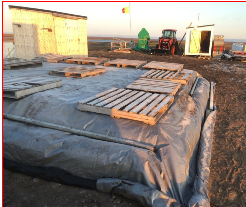
Figure 4. Fuel berm Number 2, near generator, with Jet A-1 fuel stored for the winter.
