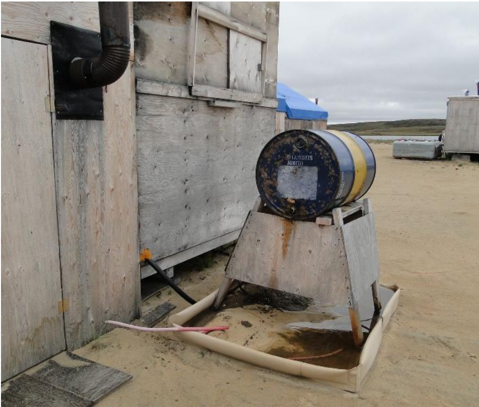
Figure 9. Barrel stand - hose has come off. Berm full of water.
