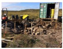
Following this excavation, done in August 2018, monitoring of the spill site was conducted on September 4<sup>th</sup> 2018. Four of the nine samples taken still exceeded the PHC fraction 3 and 4 criteria of the Environmental Guideline for Contaminated Site Remediation of the Government of Nunavut taking into account that the soil is characterized as a coarse-grained soil.
