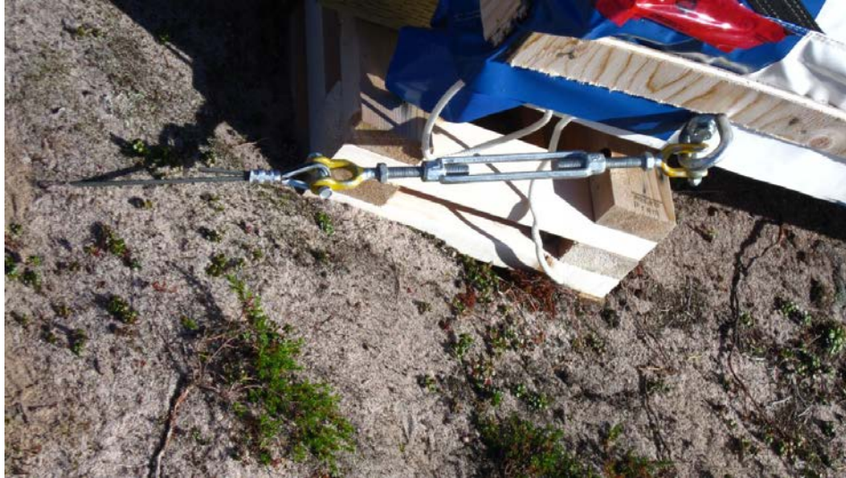
Figure 4: Photograph showing the anchoring method used to deter any further shifting of the structures during high wind events.
