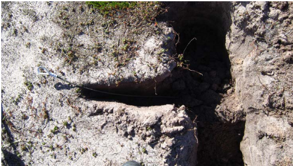
Figure 3: Photograph showing the 3 ft. deep holes where the 2 ft. long 2 x 6 were placed with the cable attached for fastening onto the tent structures.
