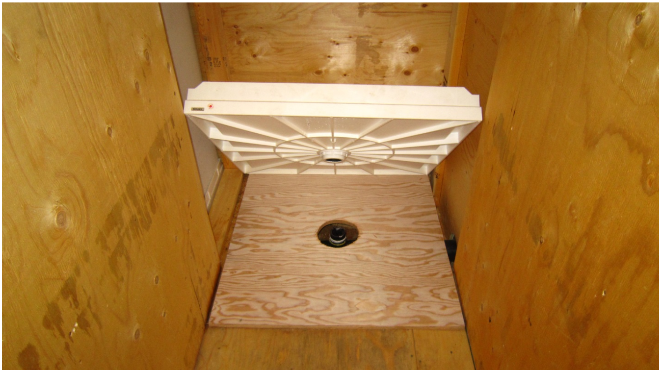
Figure 3: Photograph showing the reinforced flooring for the shower facility upgrades.
