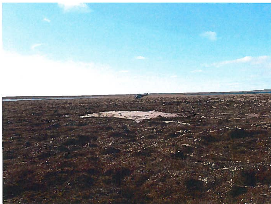
Figure 11: TUR-029, TUR-031 and TUR-033 following drilling looking west. Cuttings on the grid were directed to a natural depression in the centre of photo.
