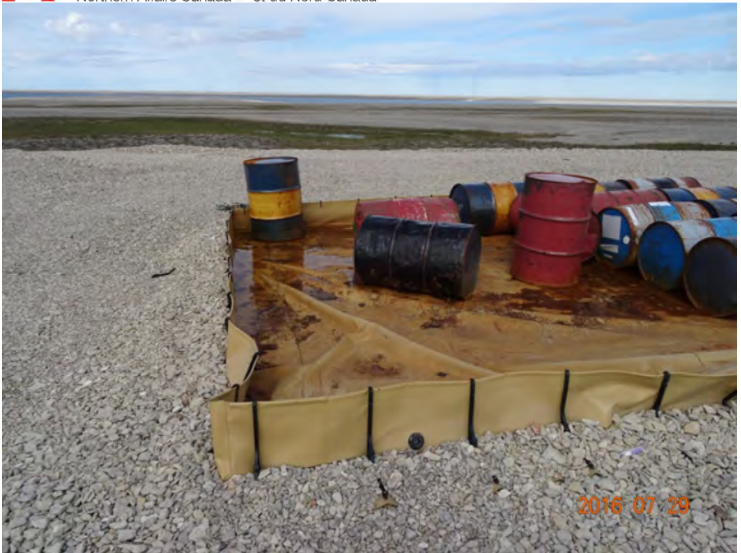
Figure 3 Roche Bay airstrip- barrel of unknown contents in secondary containment
