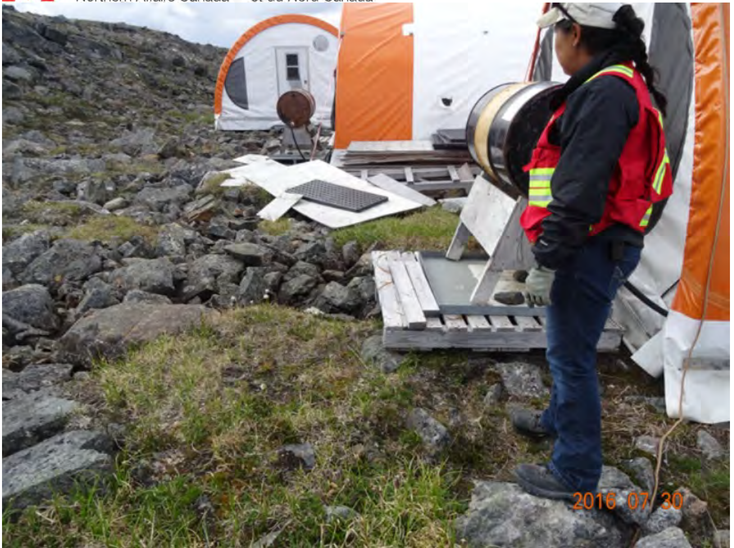
Figure 53 barrels of heating fuel on stands behind tents - hoses are all weathered and cracking
