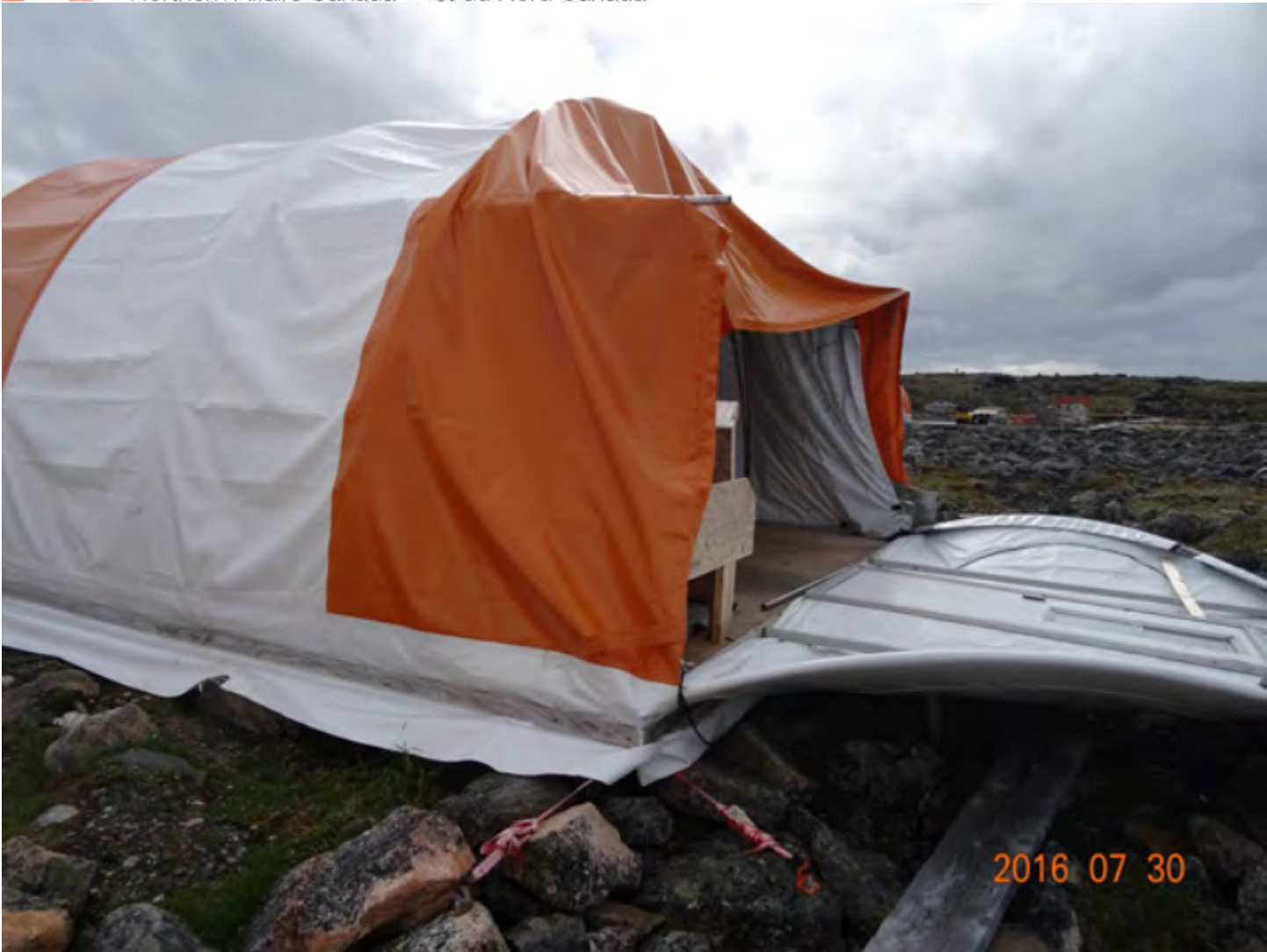
Figure 67 weather haven with end blown off
