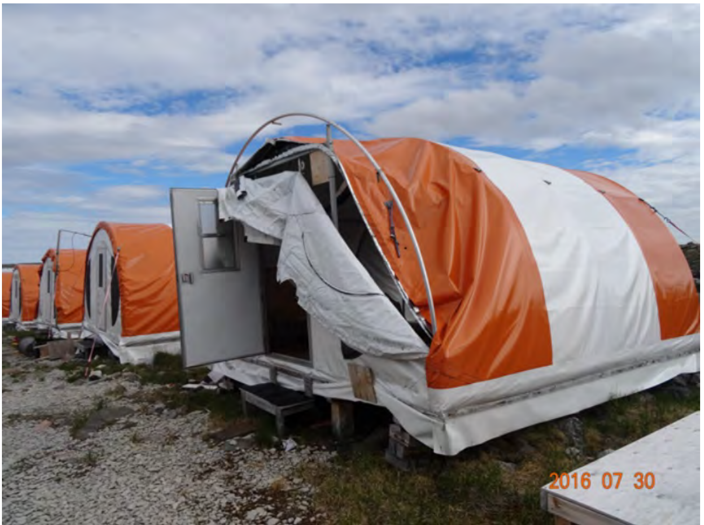
Figure 54 weather haven with wind / structural damage
