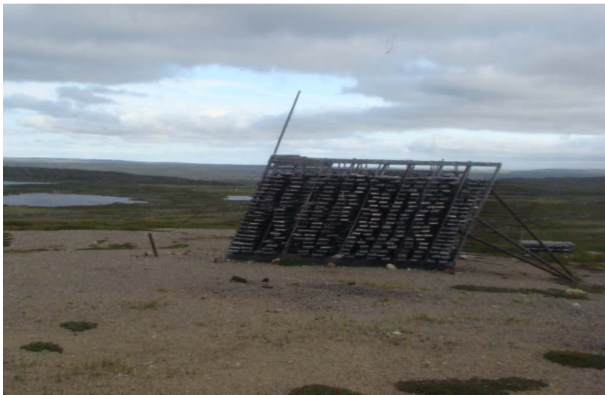
Photograph 6: View of drill core storage racks, showing significant lean to one side.
