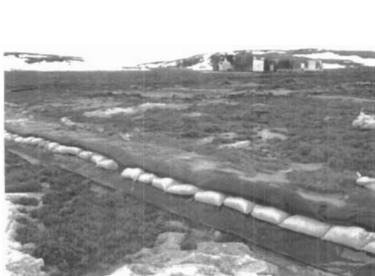
Figure 6: Retention Berm
