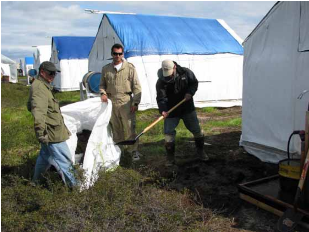
Figure 5: Excavating and bagging fuel contaminated soil.
