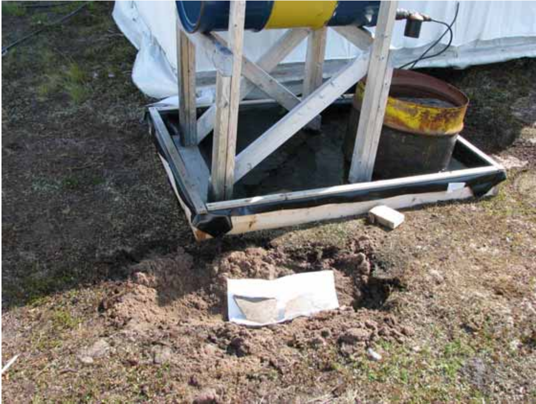
Figure 6: Excavation of fuel-contaminated soil with absorbent matting.
