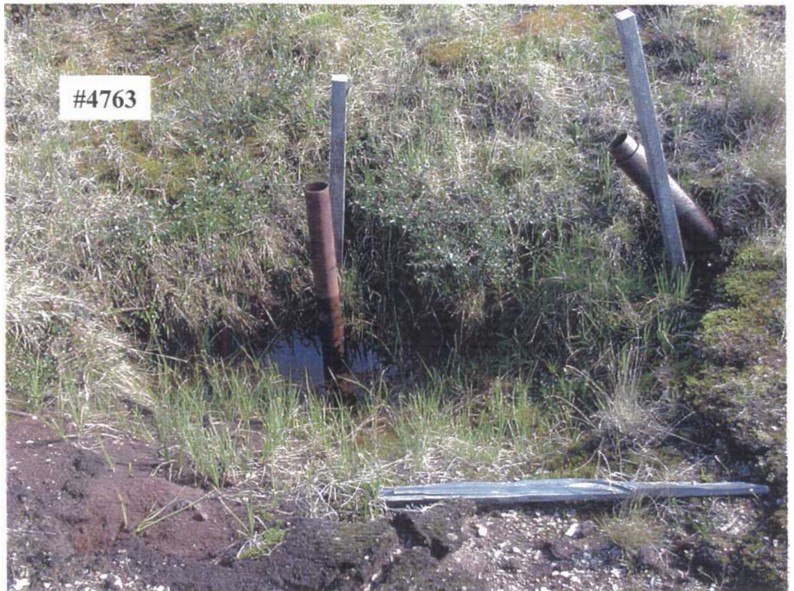
Protruding steel casing to be cut and disposed off
