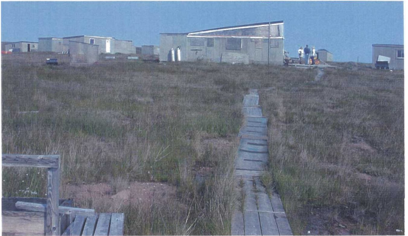
#4797: from the helicopter landing pad, looking East; kitchen/dining.
