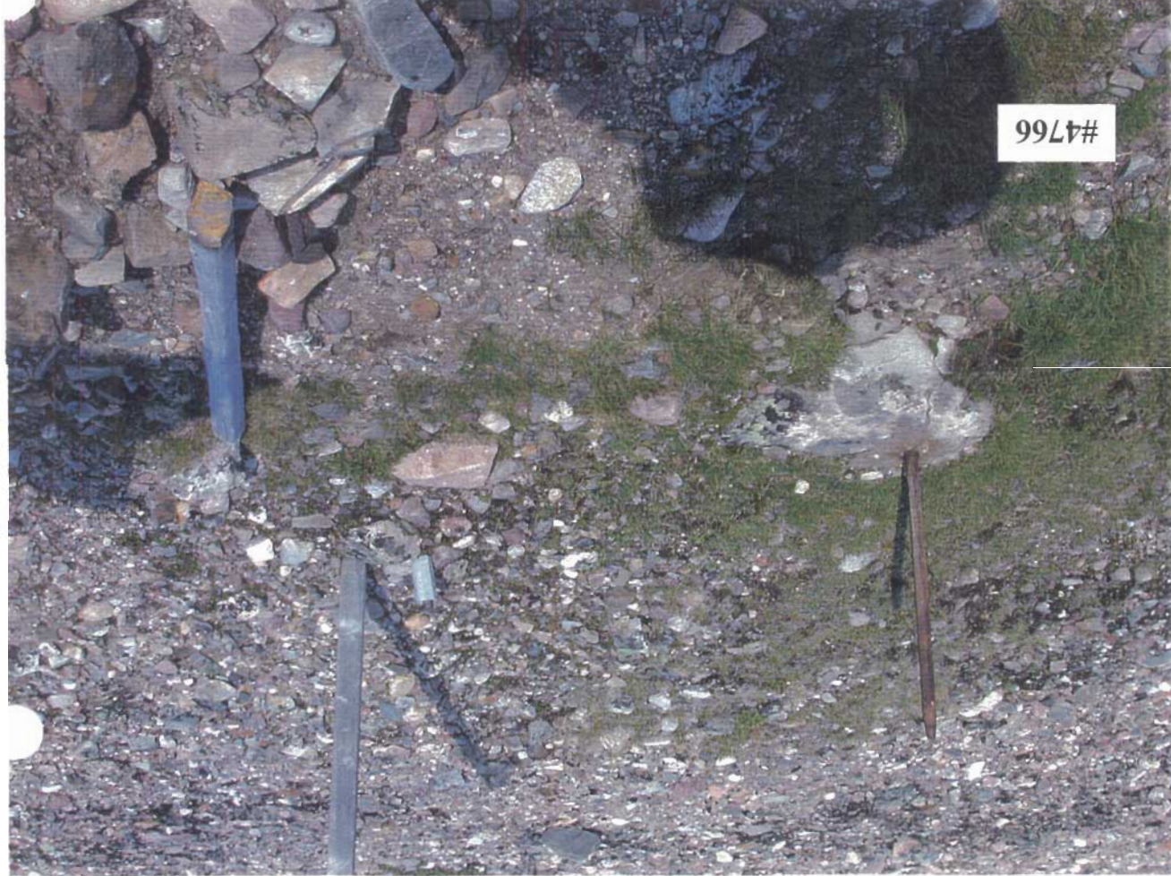
Protruding steel casing to be cut and disposed off, together with pail debris
