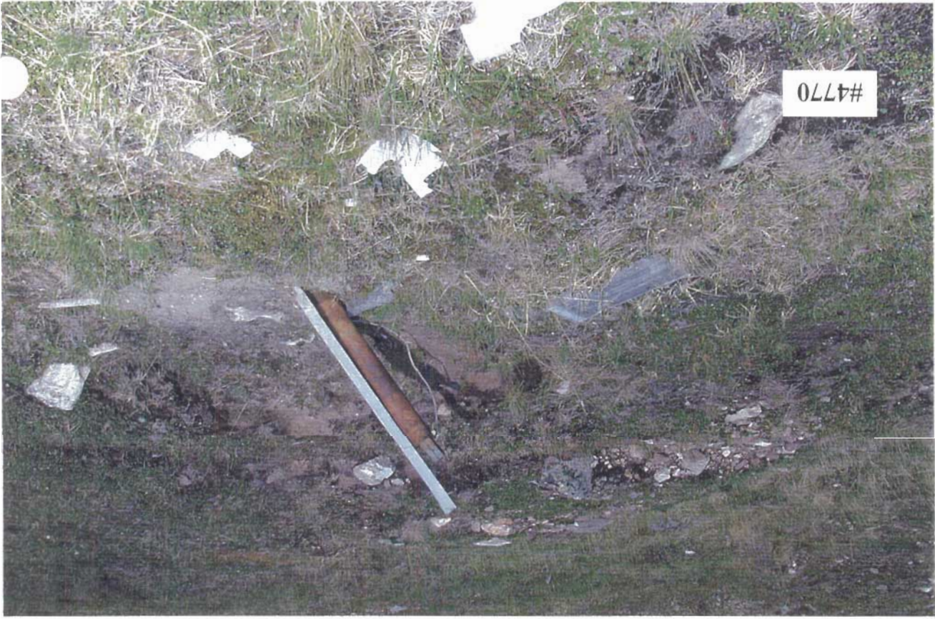
Protruding steel casing to be cut and disposed off, together with pail debris
