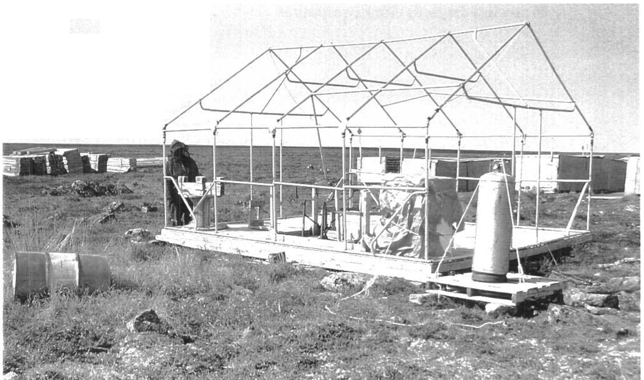
#2658: the tent frame & platform to be dismantled
