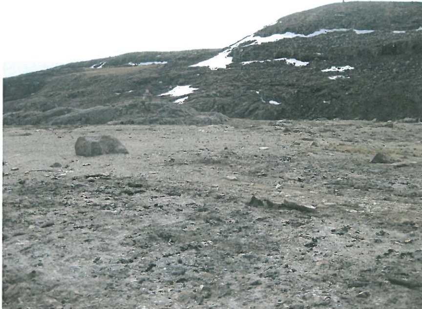
Filled In and Recontoured Kitchen and Dry Sumps
