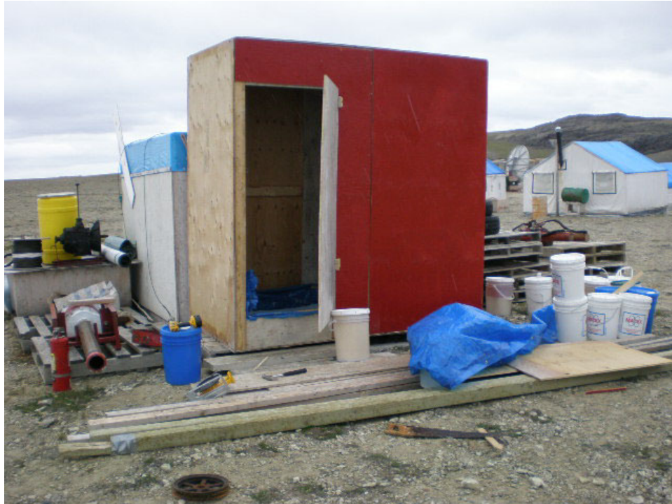
Photographs of Shed Constructed to Serve as Secondary Containment for Drilling Muds, Greases and Oils.
