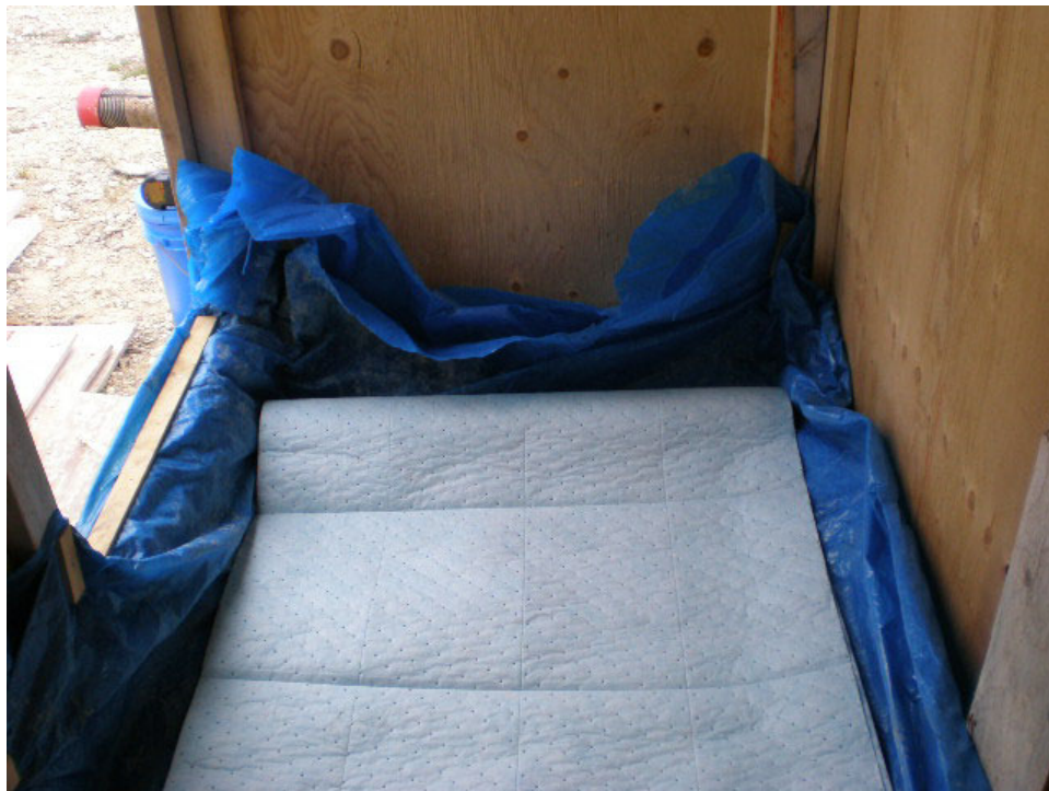
Photographs of the Interior of the Shed Built to Serve as Secondary Containment for Drilling Muds, Greases and Oils (lined with an initial layer of plastic, and topped with enviromats)
