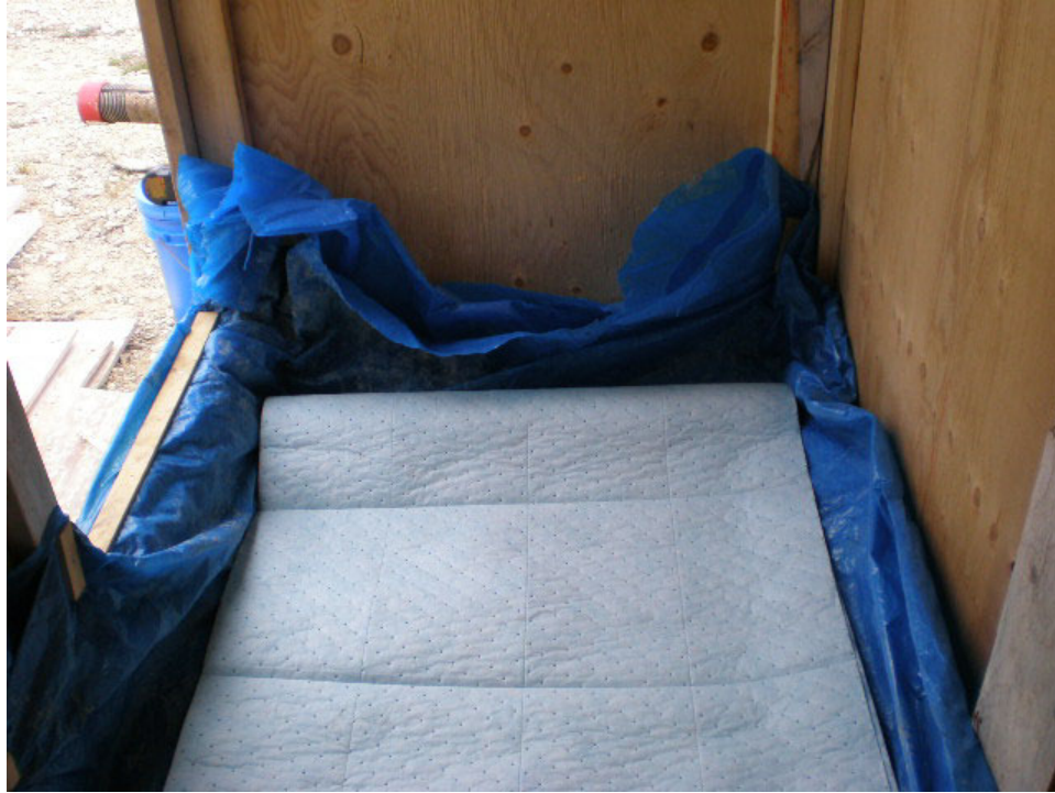
Photographs of the Interior of the Shed Built to Serve as Secondary Containment for Drilling Muds, Greases and Oils (lined with an initial layer of plastic, and topped with enviromats)
