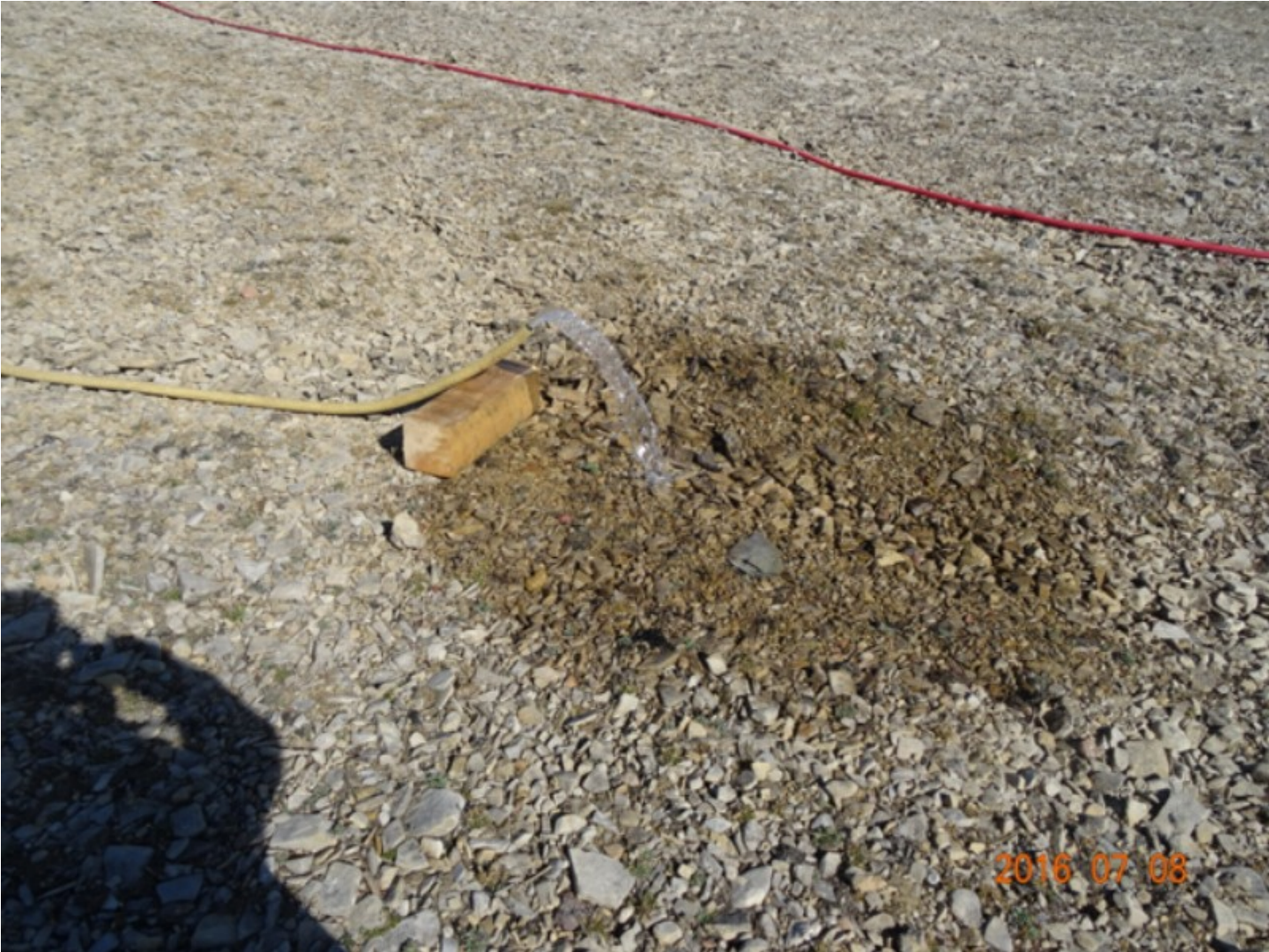
Figure 6 Return water from line at drill
