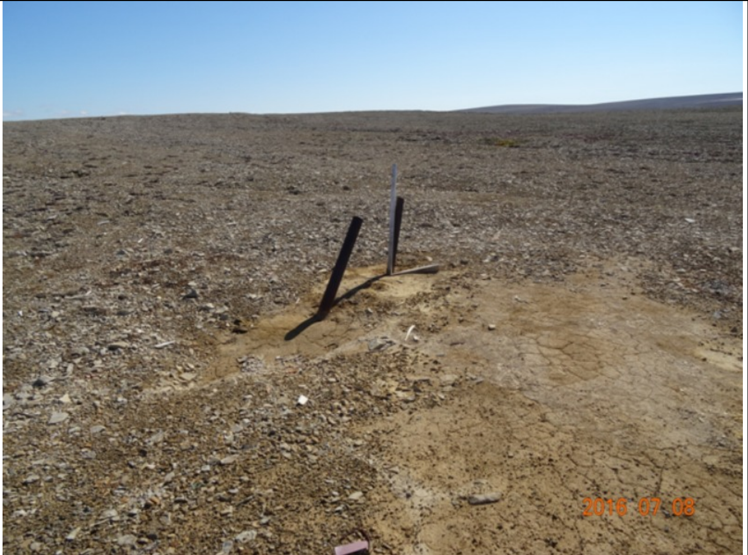
Figure 9 Legacy Site. Collars to be cut off and capped this year
