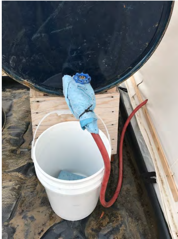
Photo 5: Tent drum in secondary containment berm. Fittings are wrapped in absorbent matting.
