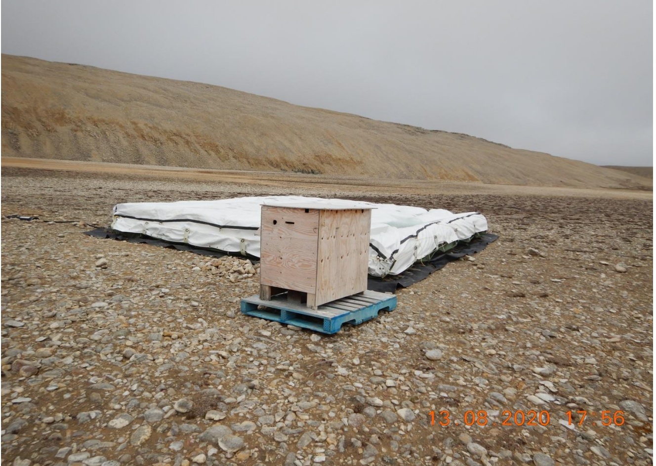
Description: Fuel Cache in secondary containment, with a cover.
