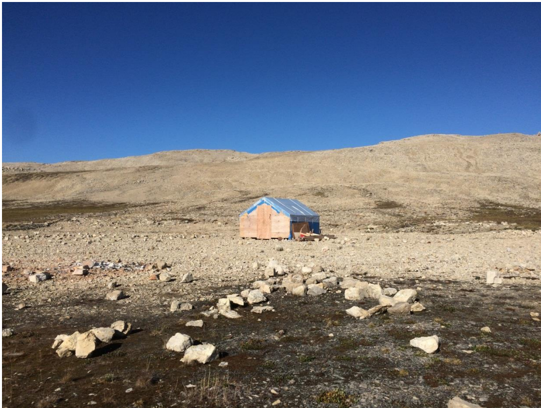
Photo 11: Aston Camp after Shutdown (looking north)
