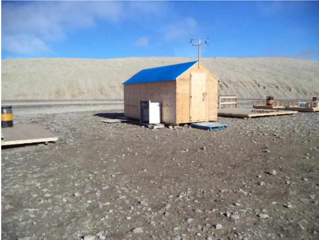
Photo 7: Storm Camp after Shutdown (looking northeast)
