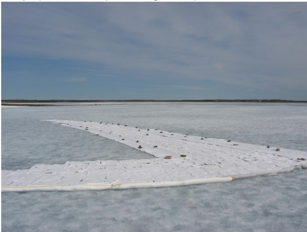
Figure 3. Hydrophobic absorbent pads covering the fuel spill area.
